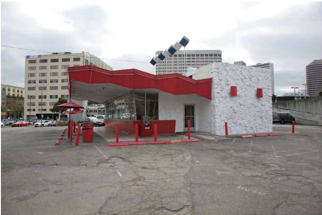
West façade, 2150 Telegraph Avenue. Source: Architecture + History, LLC, 2016.
