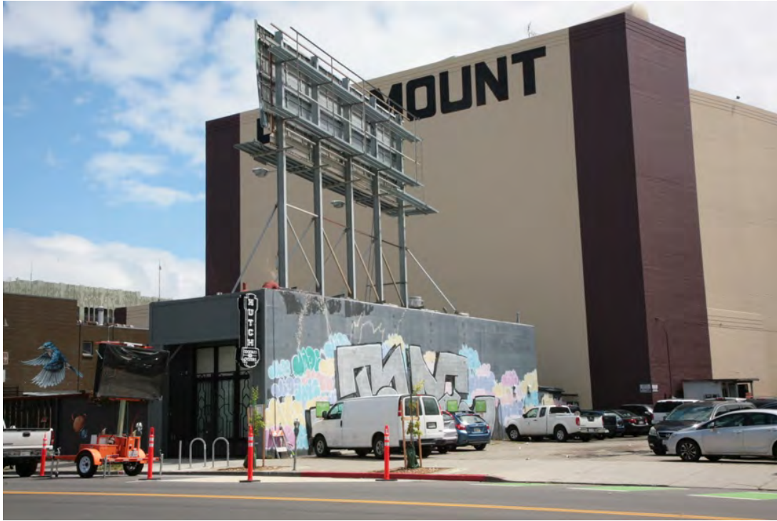
The small-scale commercial structure at 2022 Telegraph Avenue.
