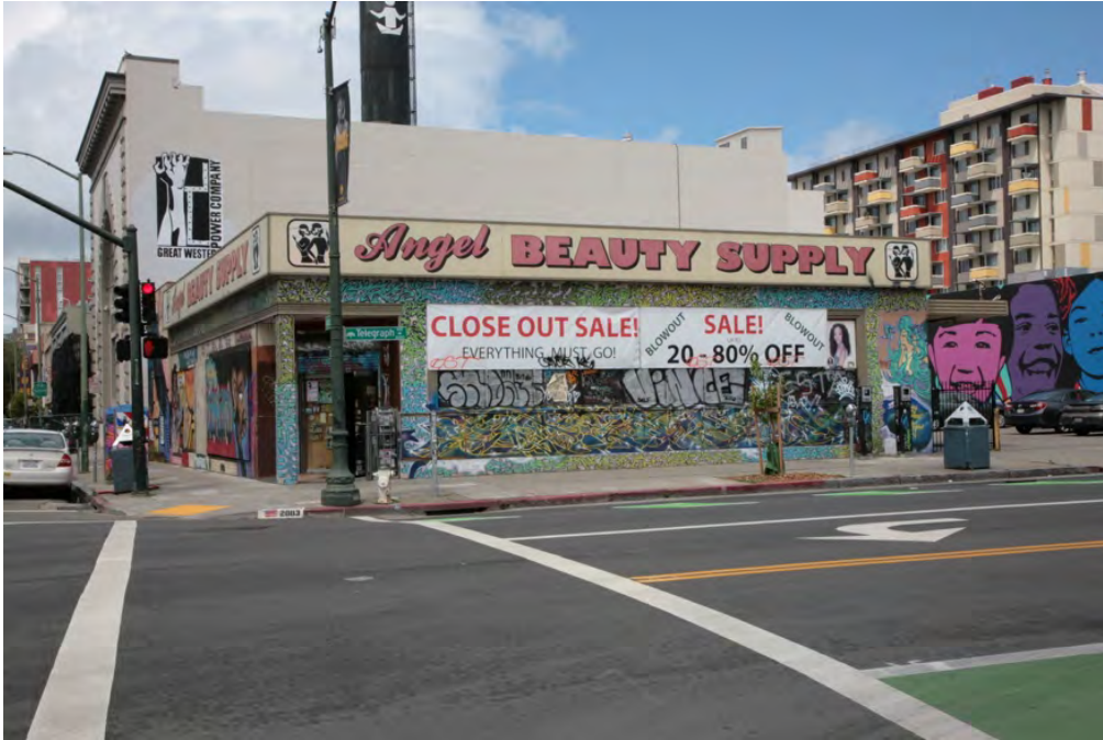
The small-scale commercial structure at 2003-09 Telegraph Avenue.
