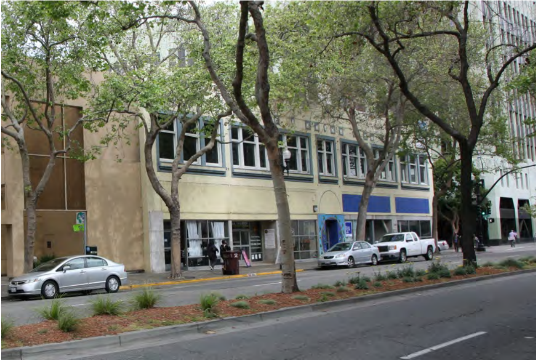
A view of the Sherman Clay Building along Broadway.
