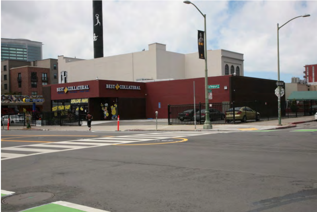
The small-scale commercial structure at 2025 Telegraph Avenue.
