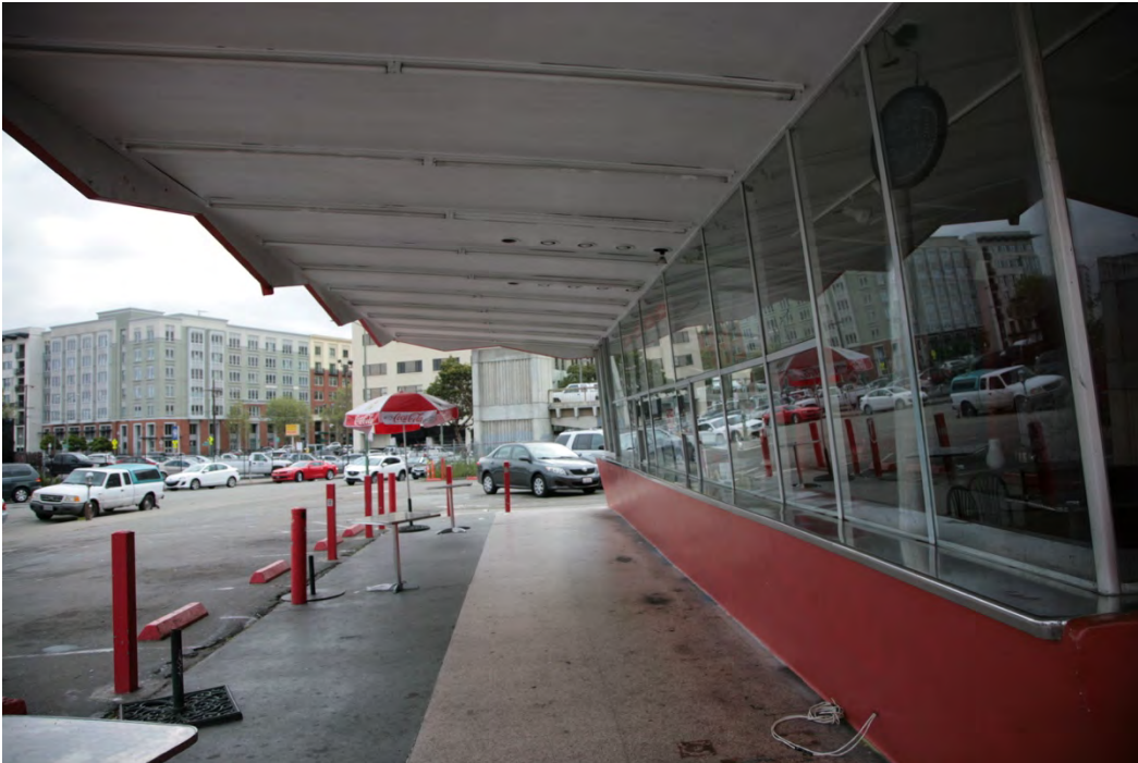
North façade detail, 2150 Telegraph Avenue. Source: Architecture + History, LLC, 2016.
