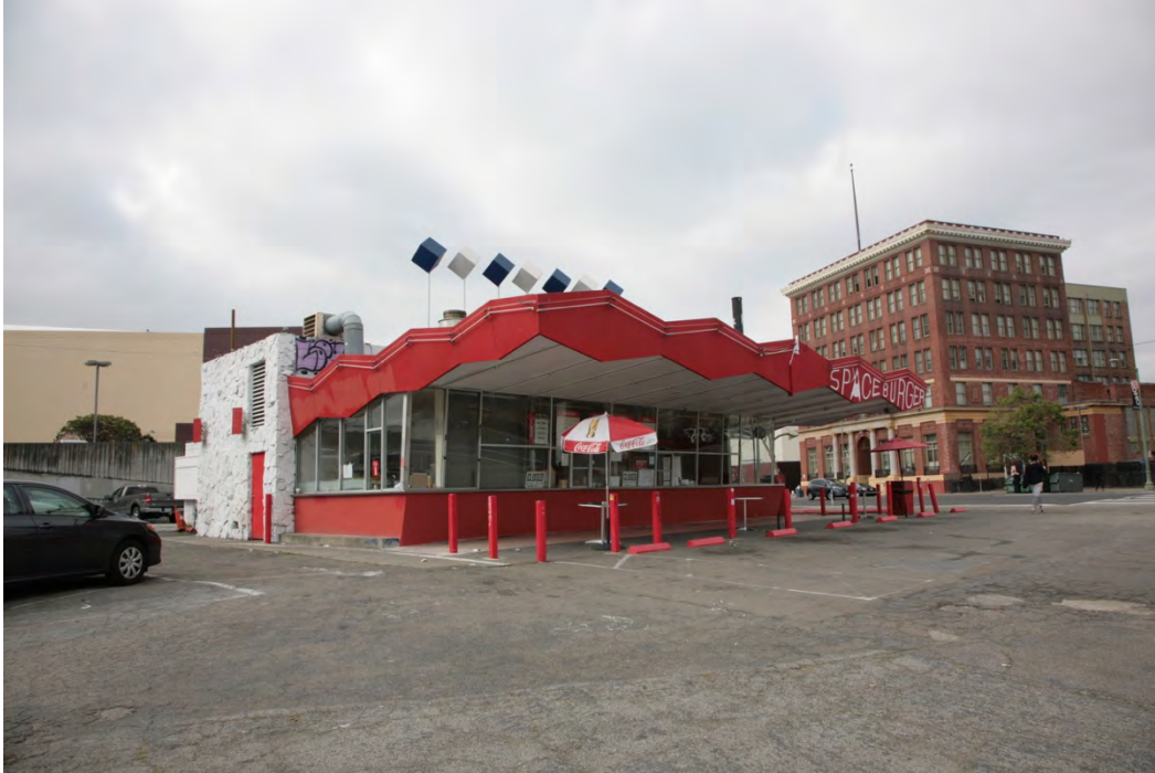
North and east façades, 2150 Telegraph Avenue. Source: Architecture + History, LLC, 2016.
