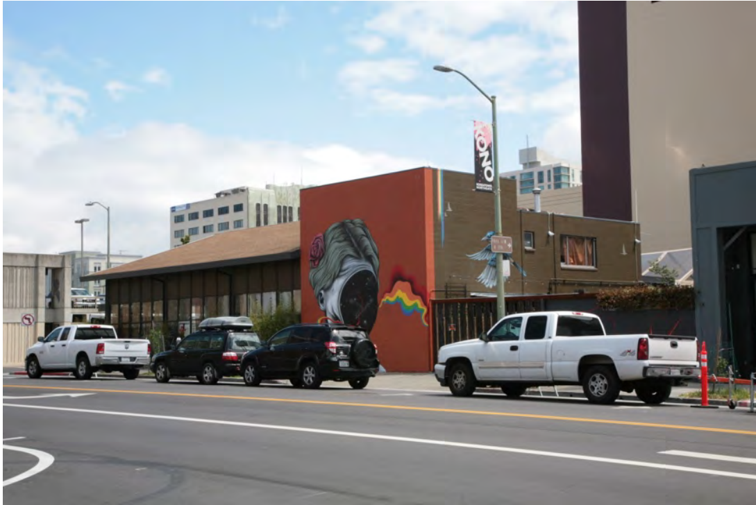
The small-scale commercial structure at 2040 Telegraph Avenue.
