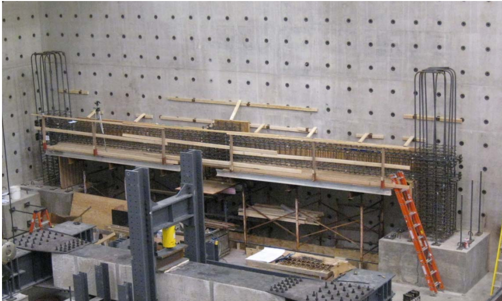
Figure 3.5 Reinforcing cage for beams and columns (SMF specimen)
