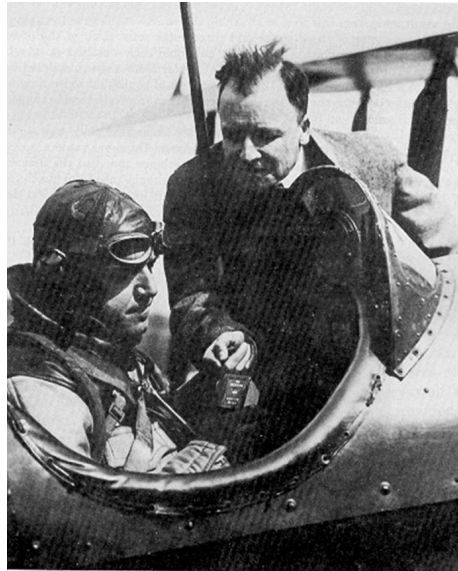
Figure 10—Dellinger explaining the vibrating-reed to MacCracken (the pilot) 66
