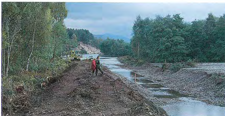
Figure 42 Excavation of the modelled flood alleviation channel on the River Spey
