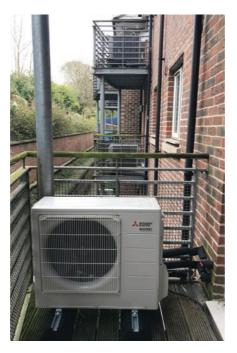
a Reading-based installation company with years of experience dealing with renewable technologies, praised the Ecodan system. "Air source heat pumps are an ideal solution that will help reduce both running costs and emissions over traditional carbon-intensive heating", comments Faulkner. "The Ecodan system is particularly suitable for properties like Bowling Court, which is in an off-gas area".
