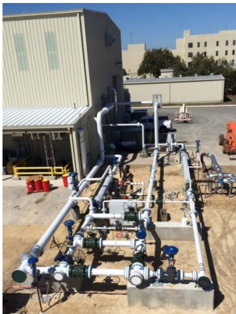
Figure 5. Pipe Loop Assembly Aerial View
