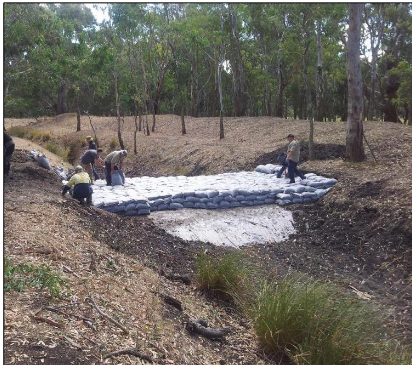
Figure 31 – The trial structure installed on 19 th March 2014 at the Brady Swamp artificial drainage outlet, to increase wetland depth and reinvigorate flows down the natural Wannon River flow path
