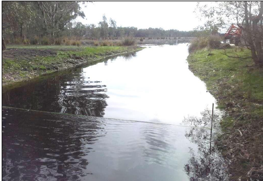
Figure 9 – Site conditions upon arrival at the site on the 26th August looking towards Gooseneck Swamp from the drain. The pegs indicate the proposed location of the sandbag weir, and the string-line was used to monitor the downstream change in channel water level in response to the works throughout the day.
