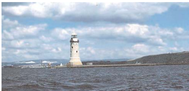
Plymouth Breakwater West Light
