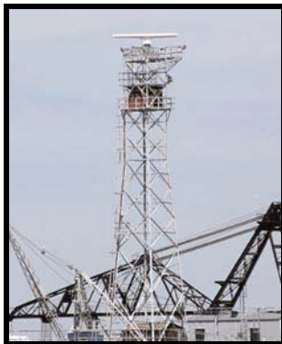
Admiralty Jetty Radar Tower
