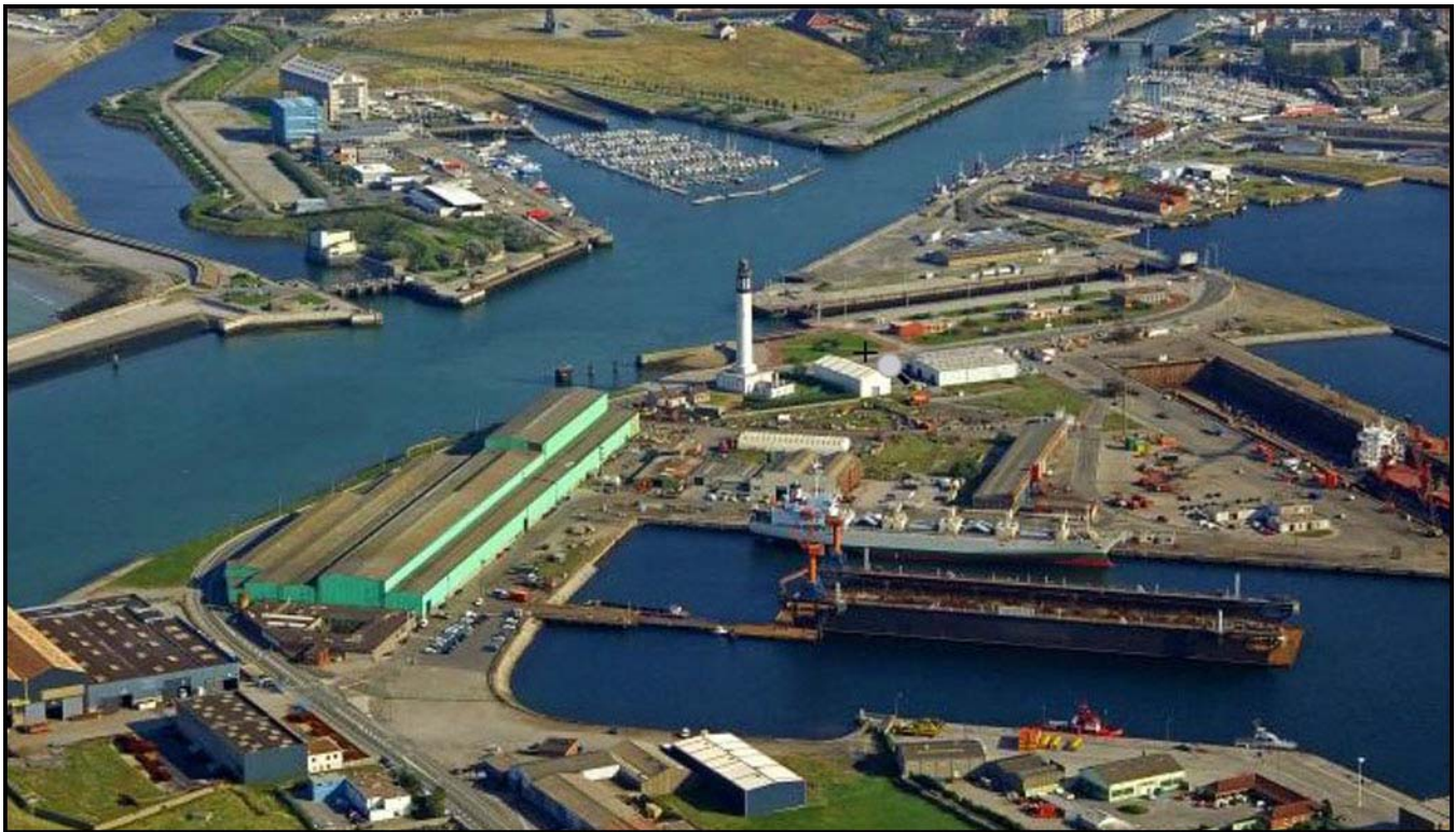
Dunkerque Harbor and Locks
