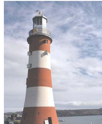
Smeaton Tower (disused)
