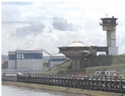
Boulogne Port Control Tower
