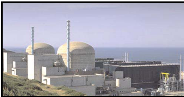
Flamanville Nuclear Power Station
