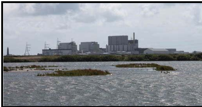
Dungeness Nuclear Power Station
