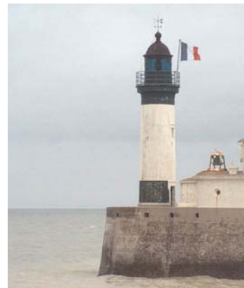
Le Treport Light (West Breakwater)
