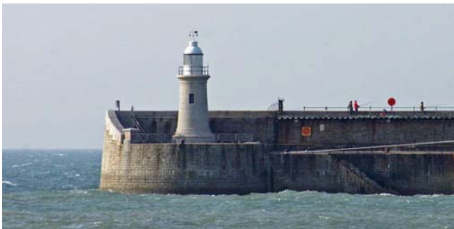
Folkestone Breakwater Light
