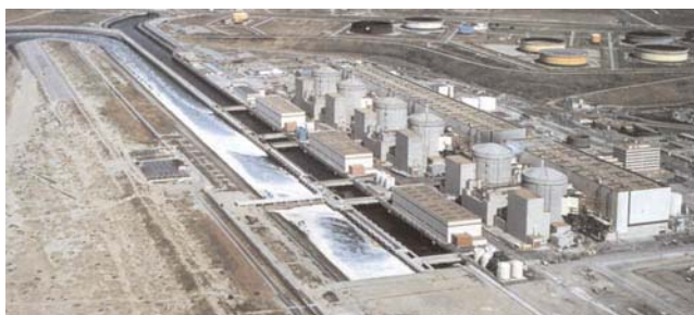
Gravelines Nuclear Power Station
