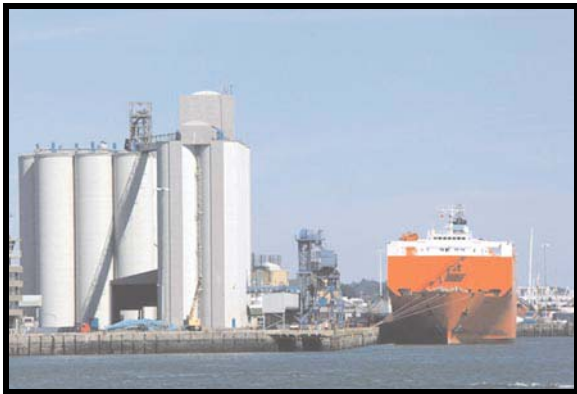
Eastern Docks Silo
