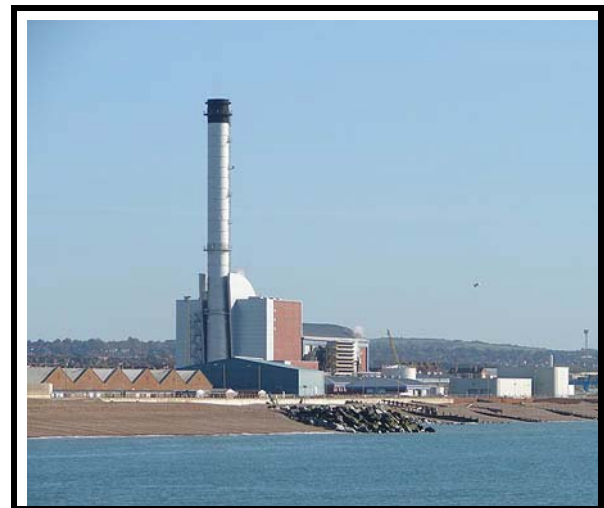
Shoreham Power Station
