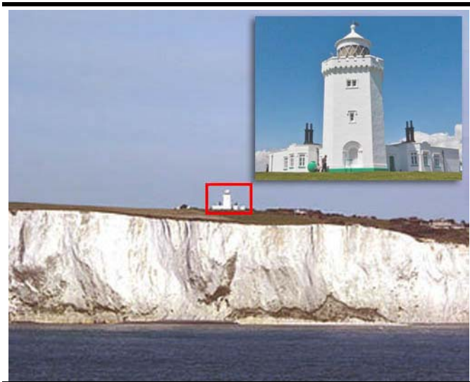
South Foreland Light Tower (disused)
