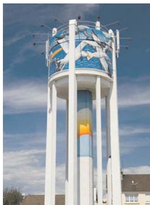
Calais—Bleriot-Plage water tower
