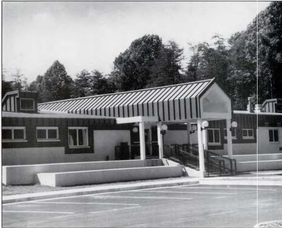
Maintenance Facility, Wheaton Regional Park
