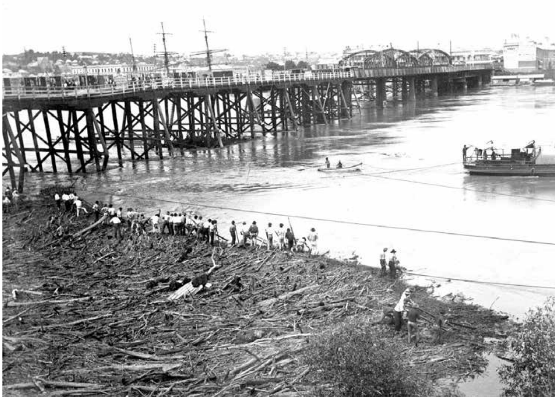
Figure 5. Debris being cleared from the temporary wooden section of the Victoria Bridge in 1896 (From author's private collection).
