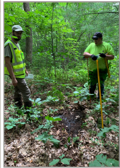
Offroad Manholes Located in GPS, marked, easements cleared
