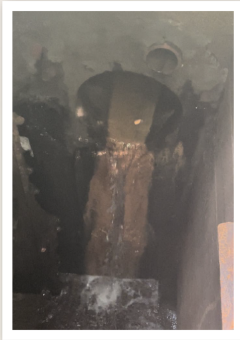
J Street Siphon inlet
