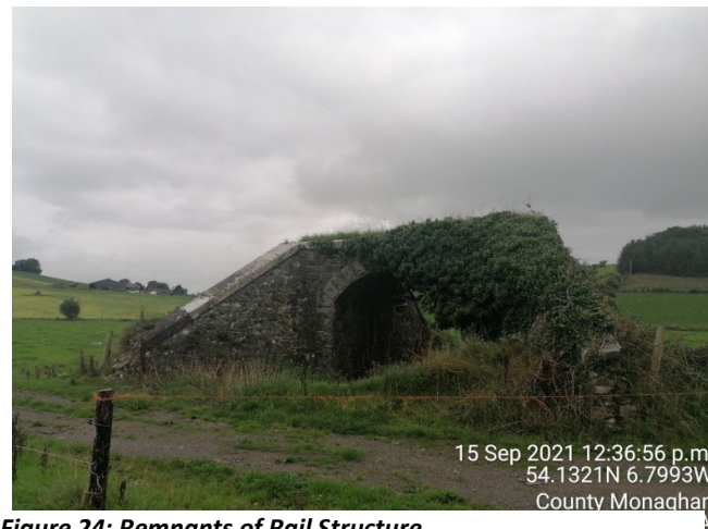
Figure 24: Remnants of Rail Structure
