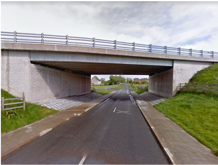
Figure 22: Mile Hill Road (L3210) Crossing under the N2
