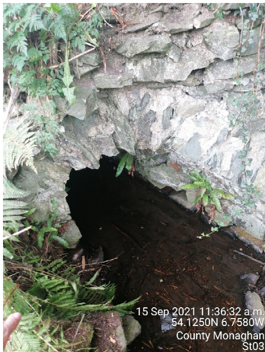
ST03 – Buried Masonry Stone Culvert
