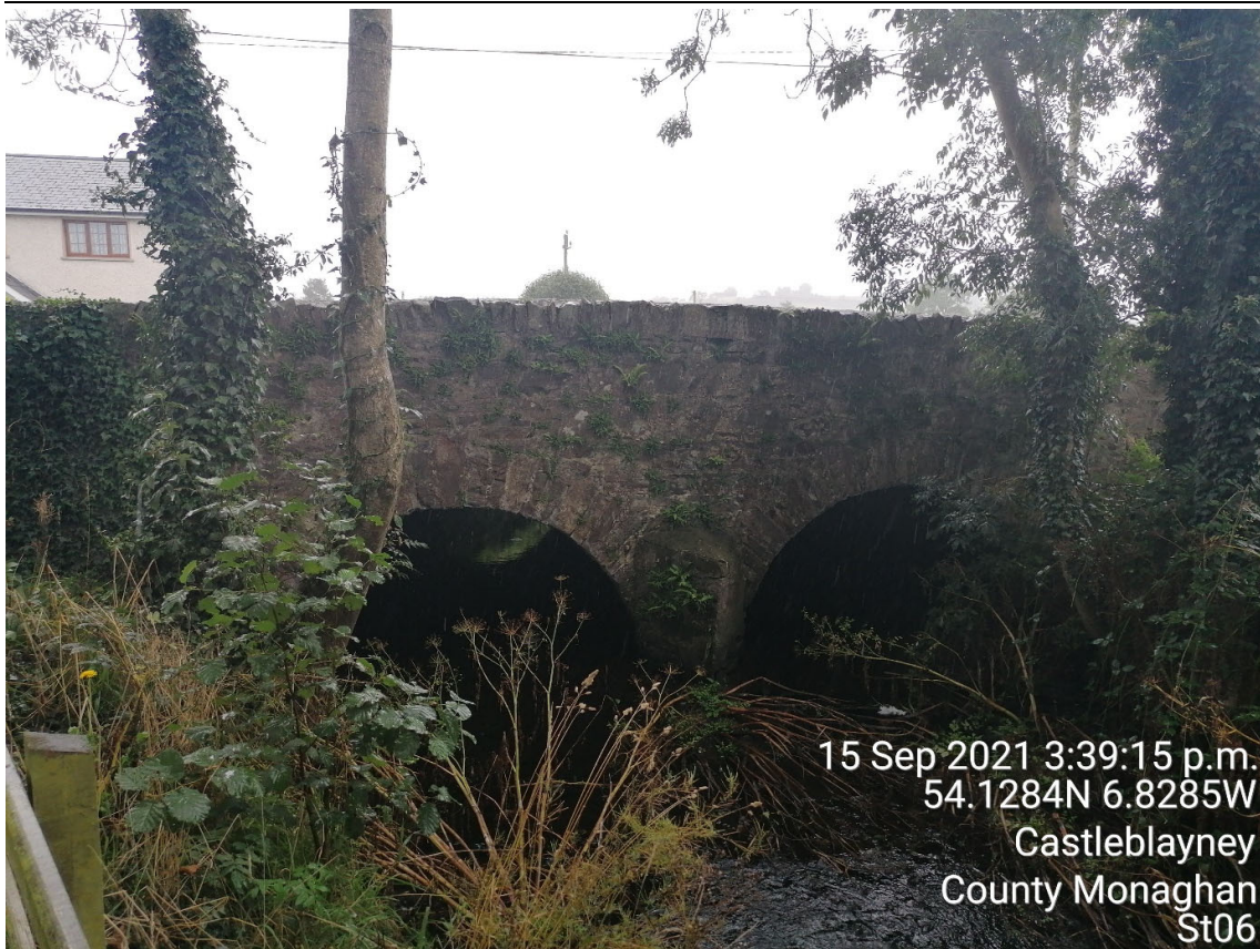
ST06 – Picture looking South at ST06
