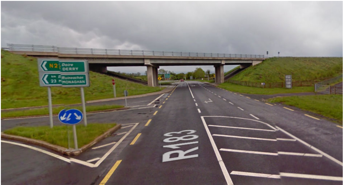
ST01 – Picture looking East at ST01
