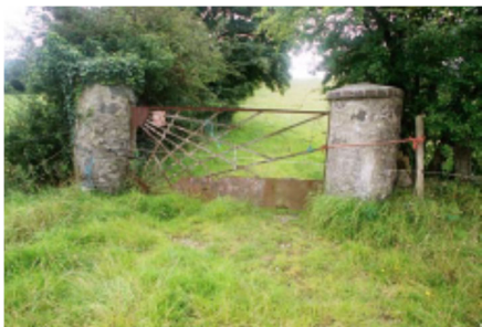
Fig 1: Cylindrical rubble stone pillars and sunburst gate on Castleblayney-Ballybay section (03511)
