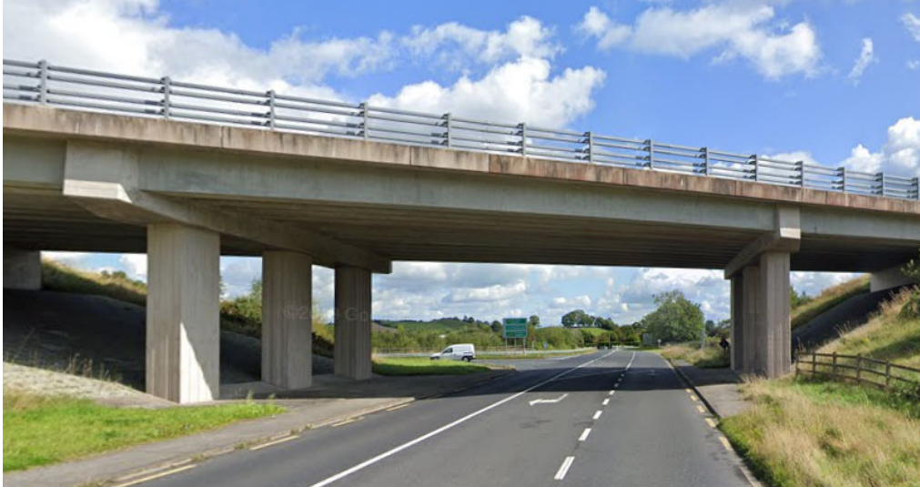
Figure 21: View of R183 Underbridge crossing of N2
