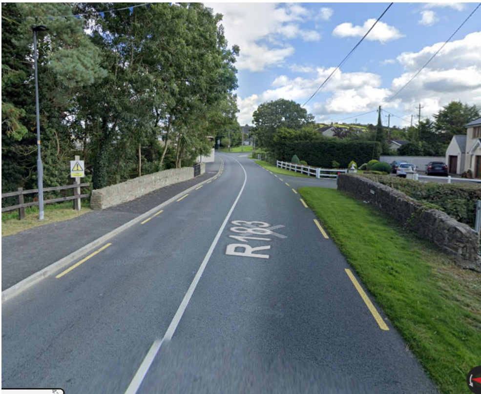
ST06 – Picture looking East at ST06
