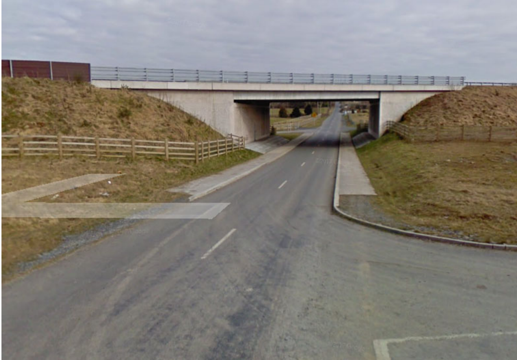
ST02 – Picture looking East at ST02
