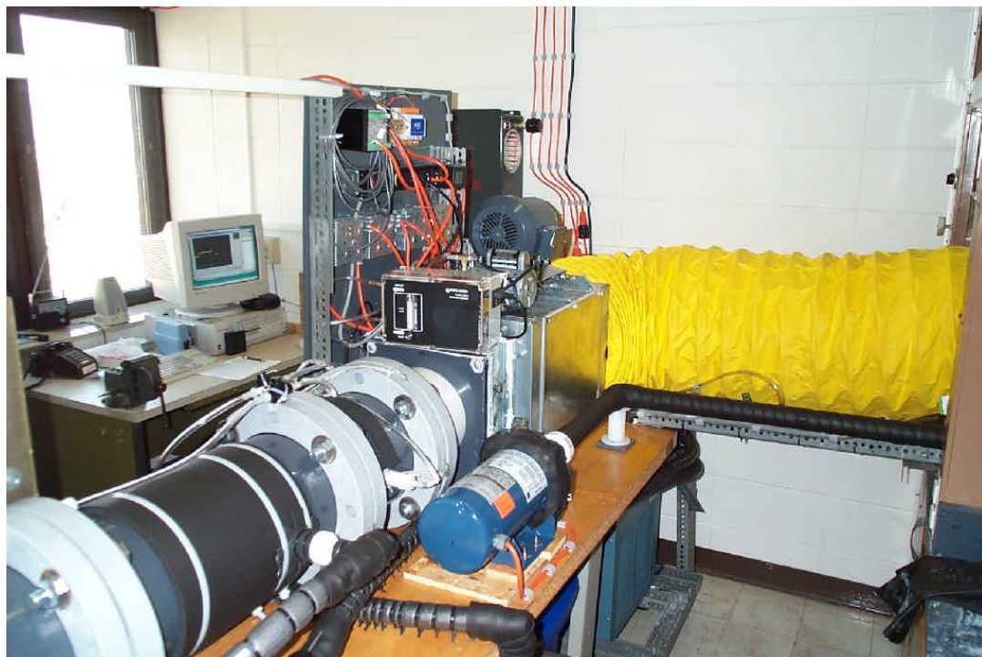
Figure F.2 View on spray unit, ozone unit, blower and exhaust duct
