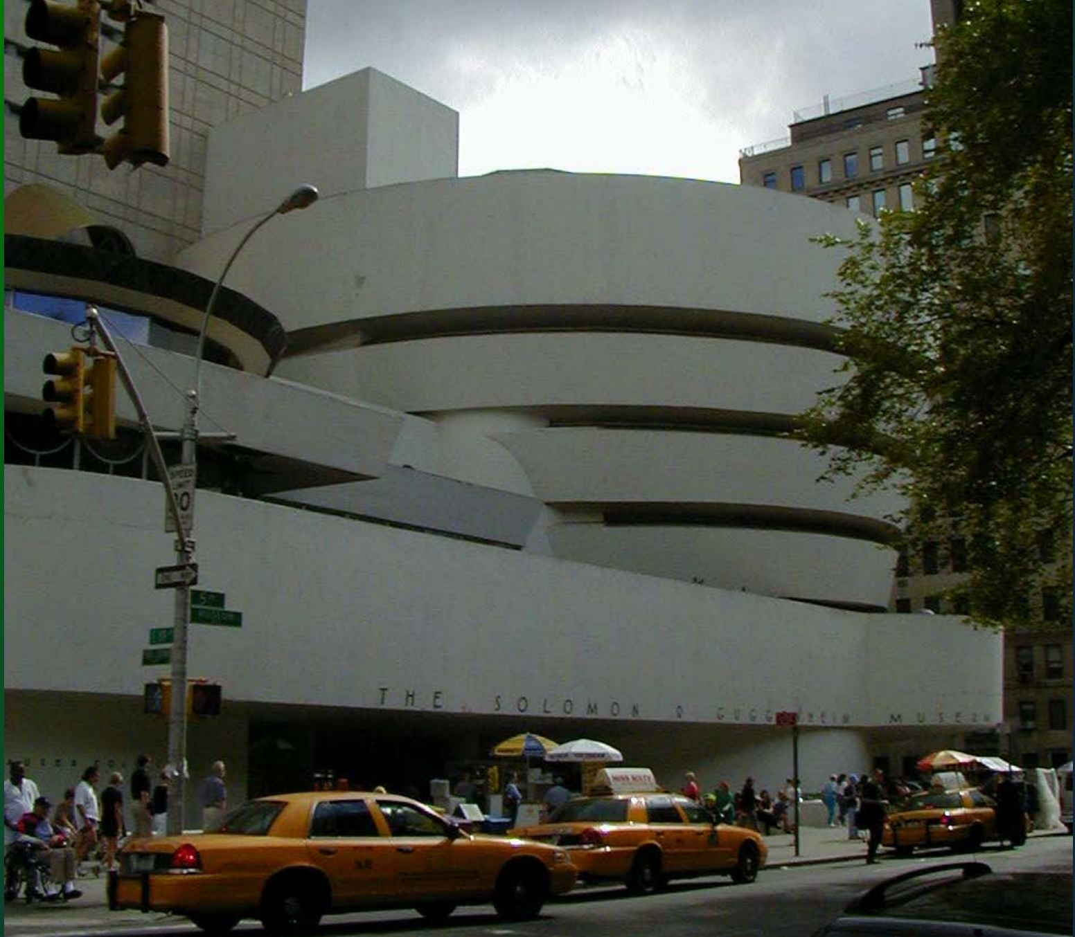
West façade on the east side of Fifth Avenue
