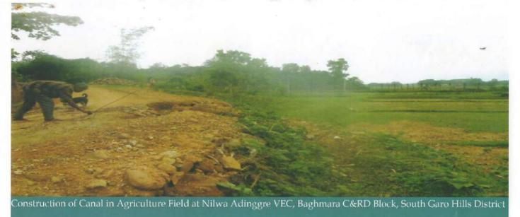
Many of the paddy fields of Nilwa Adinggre VEC lies below a hillock. During the rainy season ,excessive rain water flows down the hillock and flooded the paddy fields causing extensive damaged. The canal was constructed to control the overflow of rain water and soil erosion thereby prevent the agricultural land from being damaged. Therefore, it has tremendously helped the farmers of that area and at the same time channelise the water when required for irrigation purposes.
