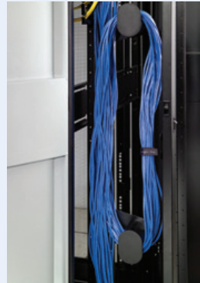
Vertical cable management channel
