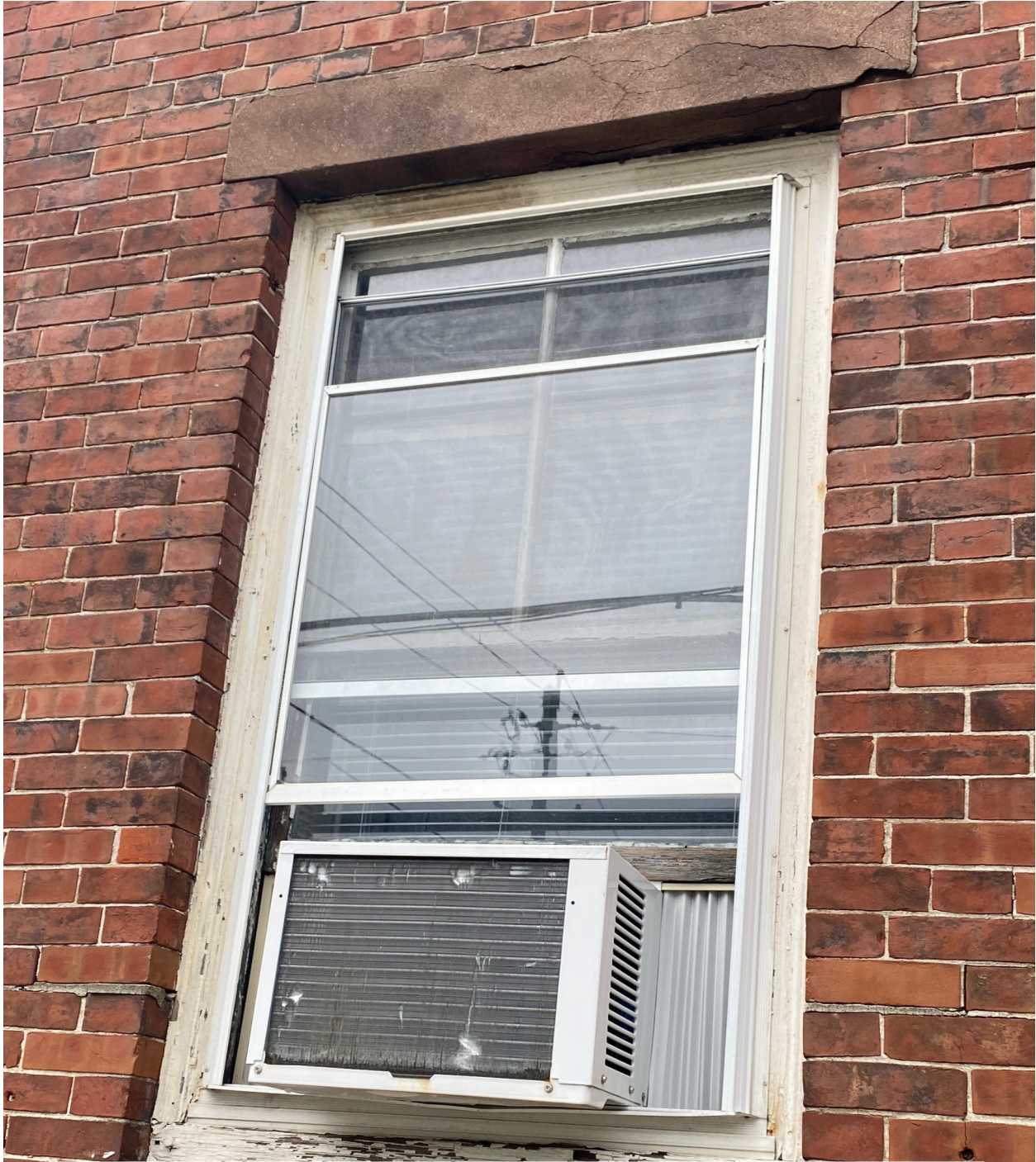
example of existing window
