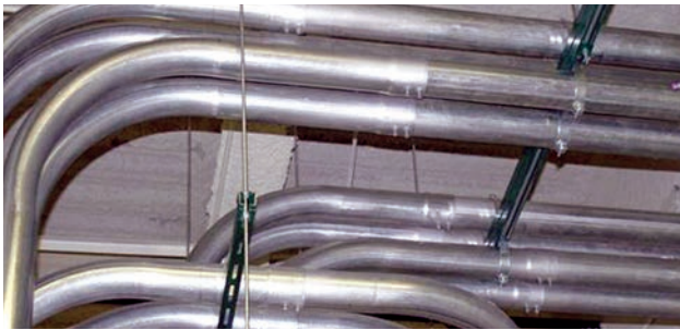
Faster EMT Installations
