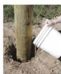
Pour mixture into prepared hole with pole
