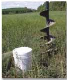
Prepare hole for pole
