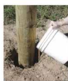
Pour mixture into prepared hole with pole
