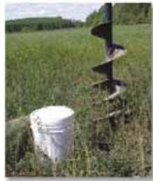
Prepare hole for pole
