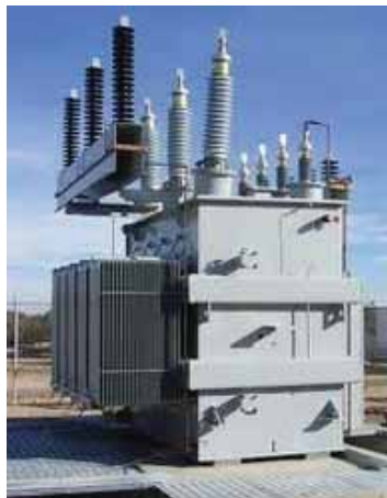
Station Class Tx Refurbs
