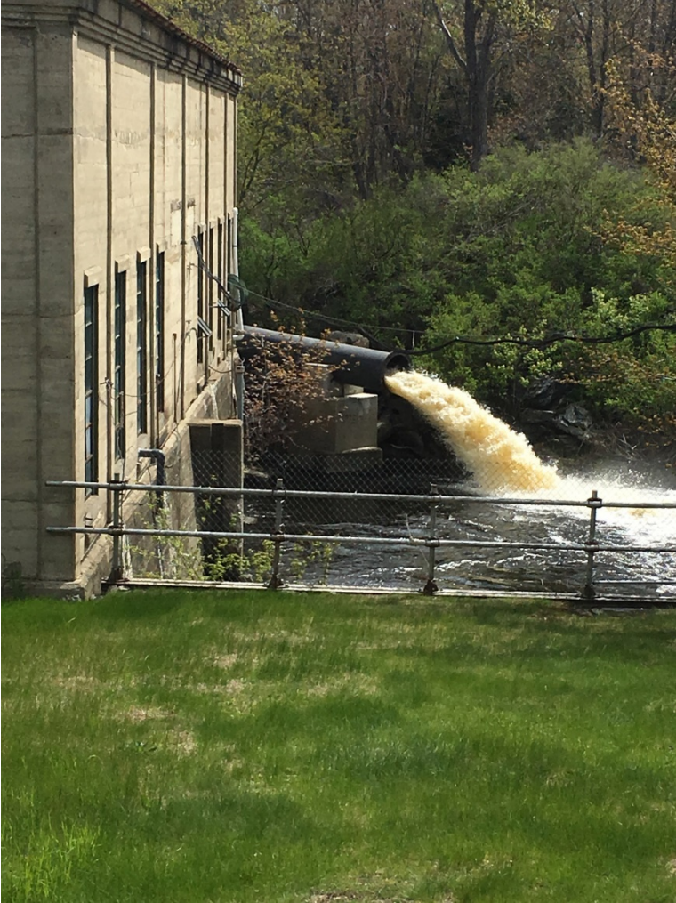
FIGURE 15. PROJECT POWERHOUSE A AND DOWNSTREAM FISH PASSAGE FACILITY – STILLWATER PROJECT
