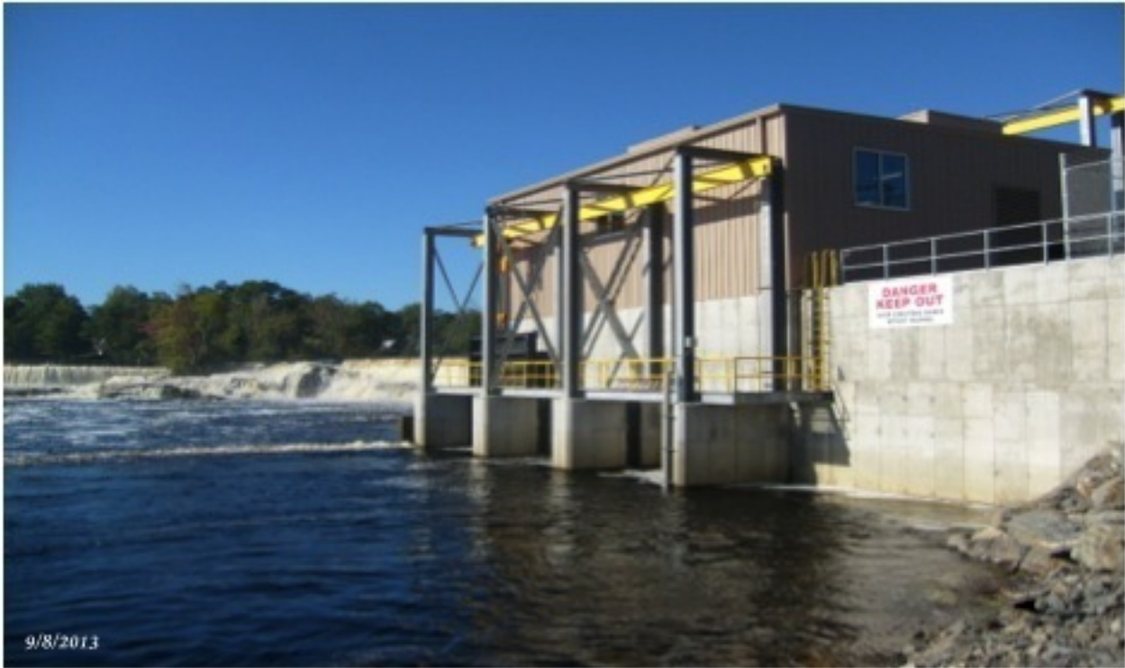
FIGURE 16. PROJECT POWERHOUSE B – STILLWATER PROJECT
