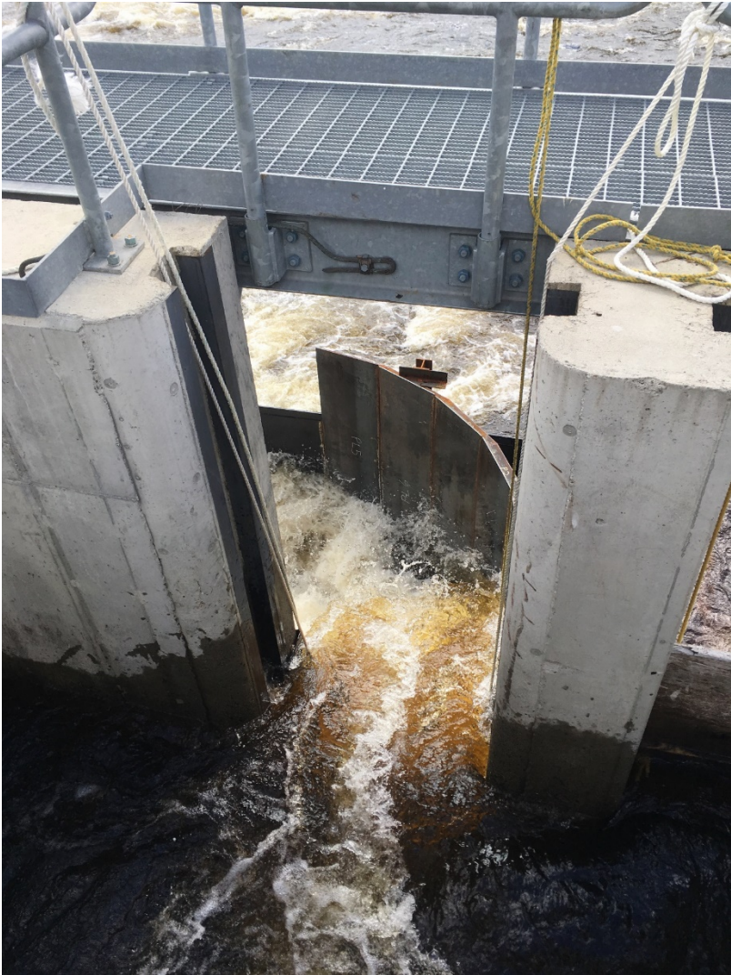
FIGURE 10. PROJECT DOWNSTREAM FISH PASSAGE FACILITY – ORONO PROJECT
