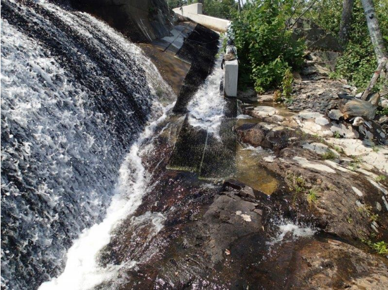
FIGURE 18. PROJECT UPSTREAM EEL PASSAGE FACILITY – STILLWATER PROJECT
