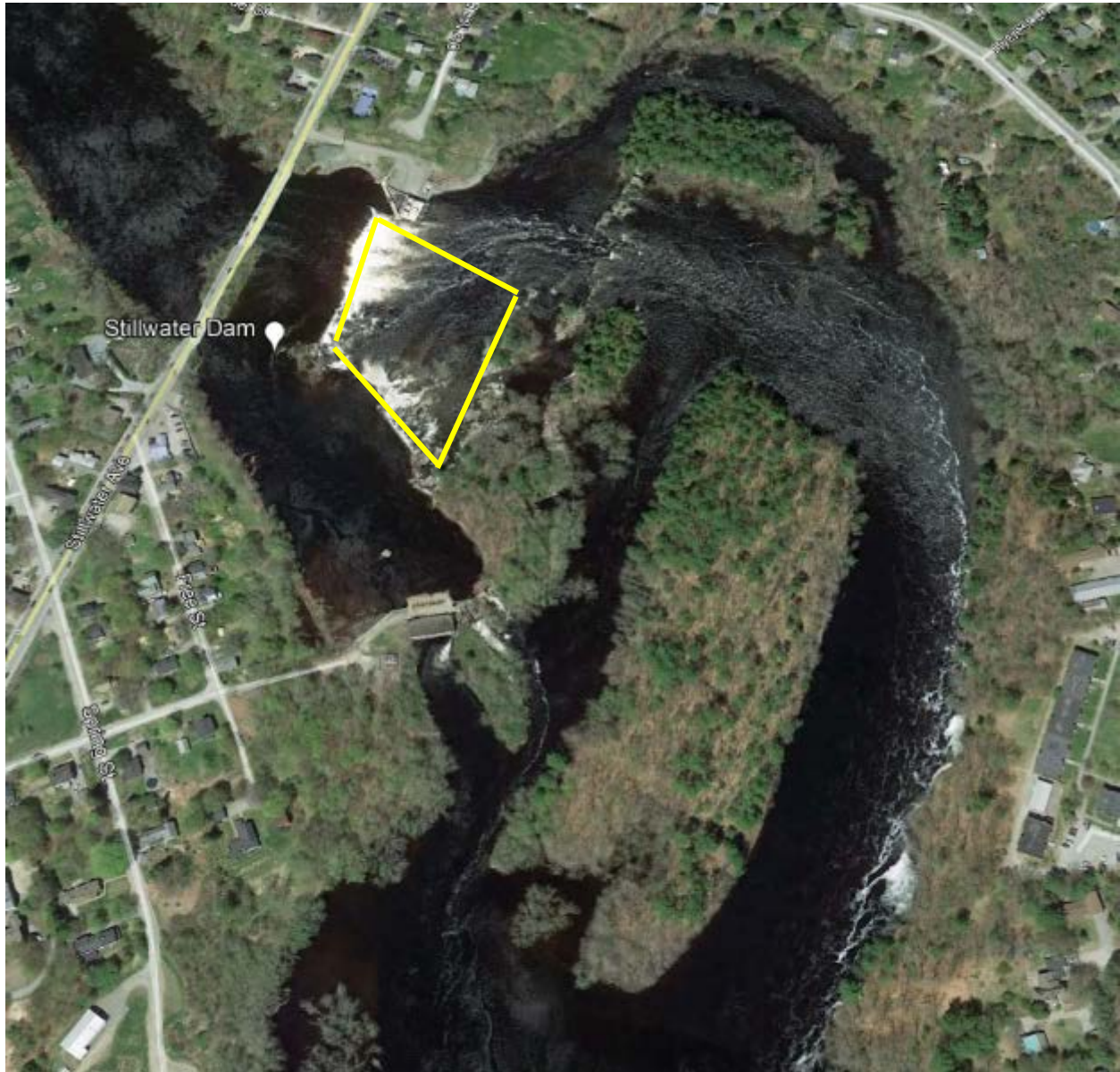
FIGURE 25. ZONE 3 – STILLWATER DAM BYPASS REACH
