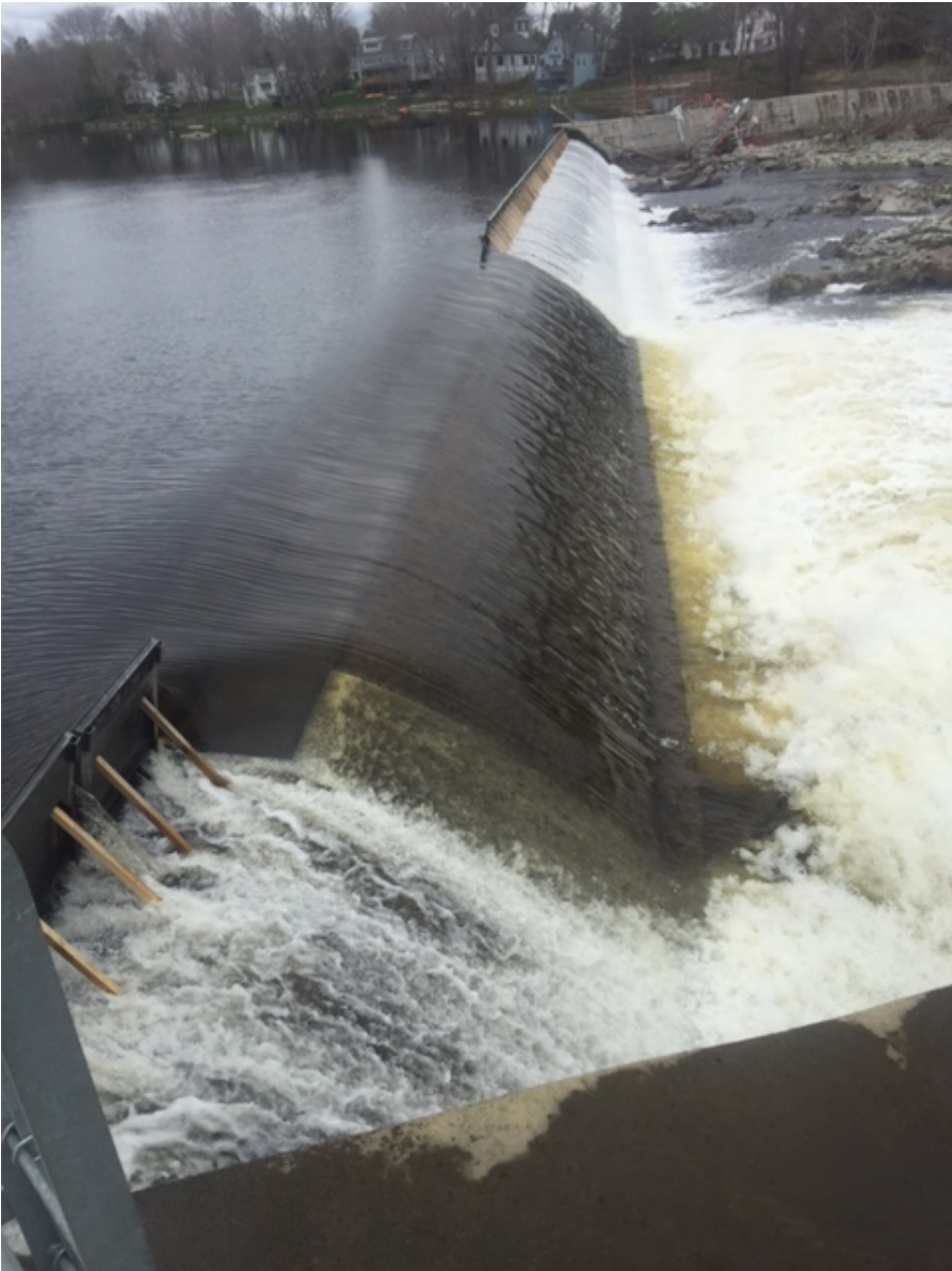
FIGURE 5. PROJECT SPILLWAY – ORONO PROJECT
