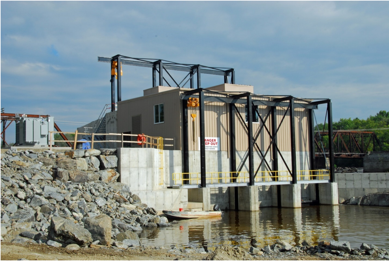
FIGURE 7. PROJECT POWERHOUSE B – ORONO PROJECT
