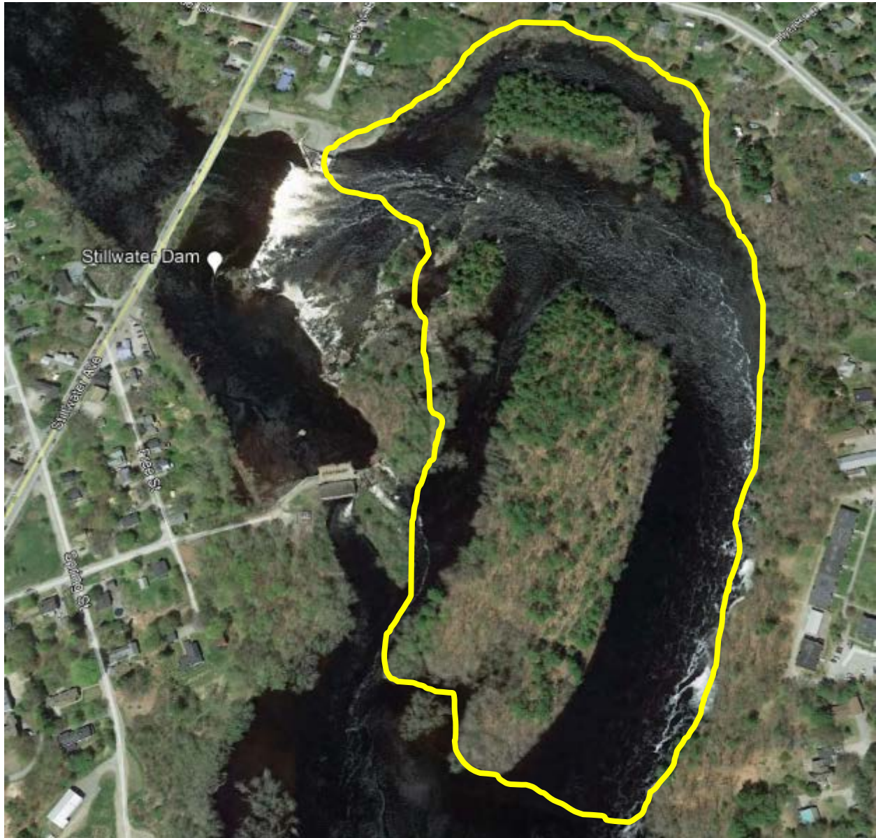
FIGURE 26. ZONE 4 – STILLWATER POWERHOUSE B TAILRACE
