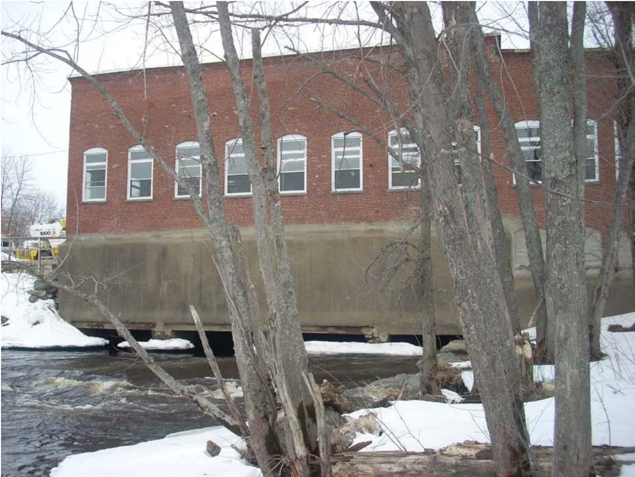
FIGURE 6. PROJECT POWERHOUSE A – ORONO PROJECT
