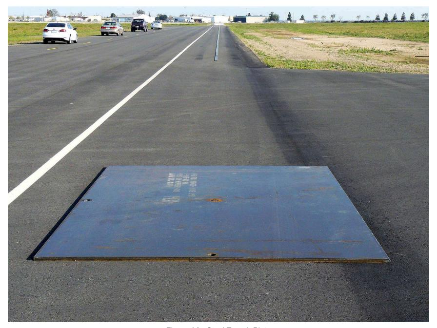
Figure A9. Steel Trench Plate
