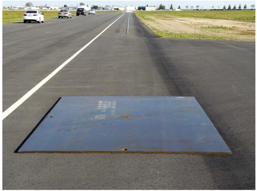
Figure A9. Steel Trench Plate
