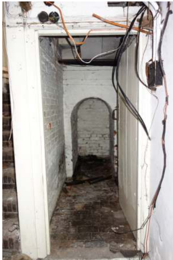
4.34: Store beside secondary stairs up from lower ground floor
