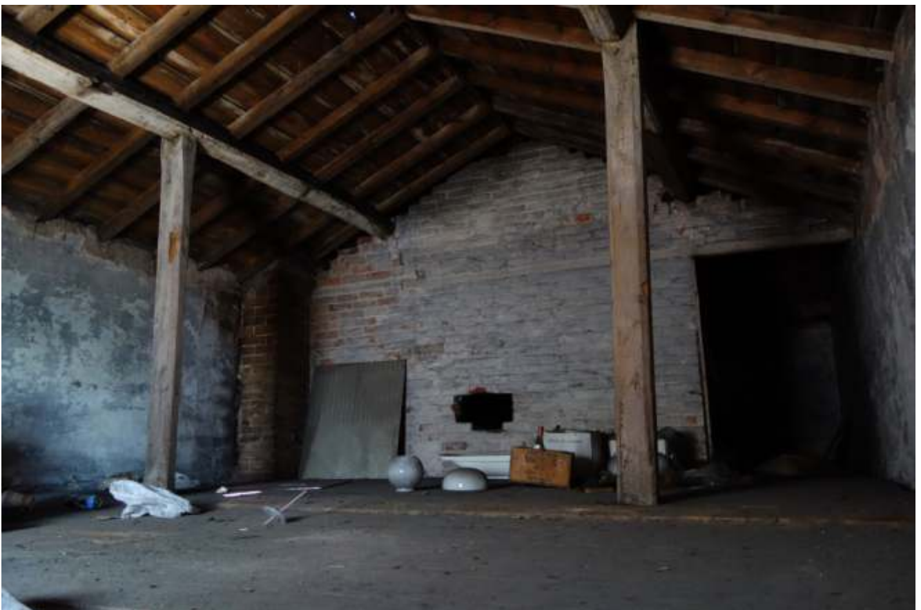
4.17: First floor of stables
