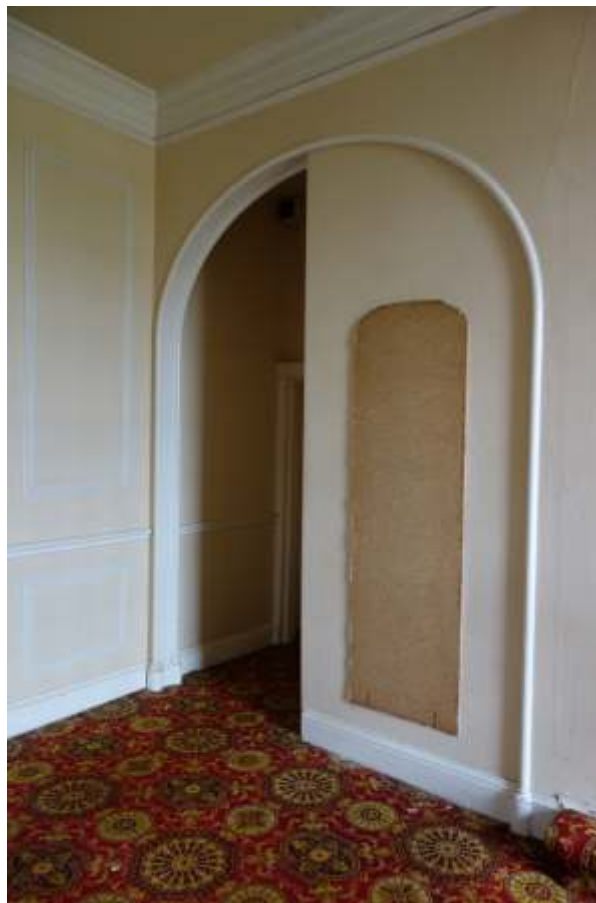
4.48: First floor landing to secondary stairs
