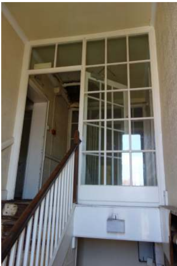
4.60: Second floor landing to secondary staircase
