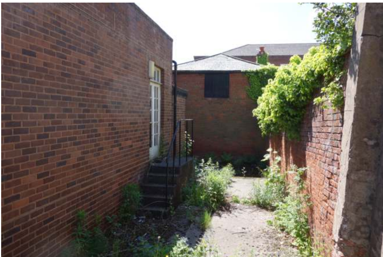
4.10: Side wall of coach house looking towards stables
