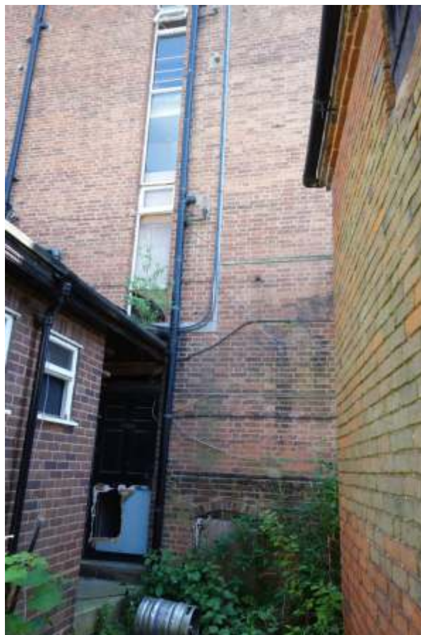
4.12: Rear wall of coach house and side wall of house
