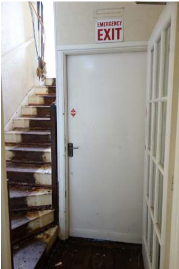
4.57: First floor lobby on secondary staircase
