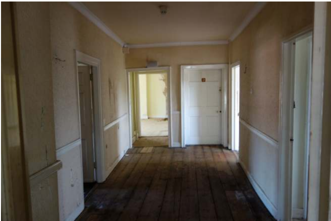
4.62: Second floor corridor
