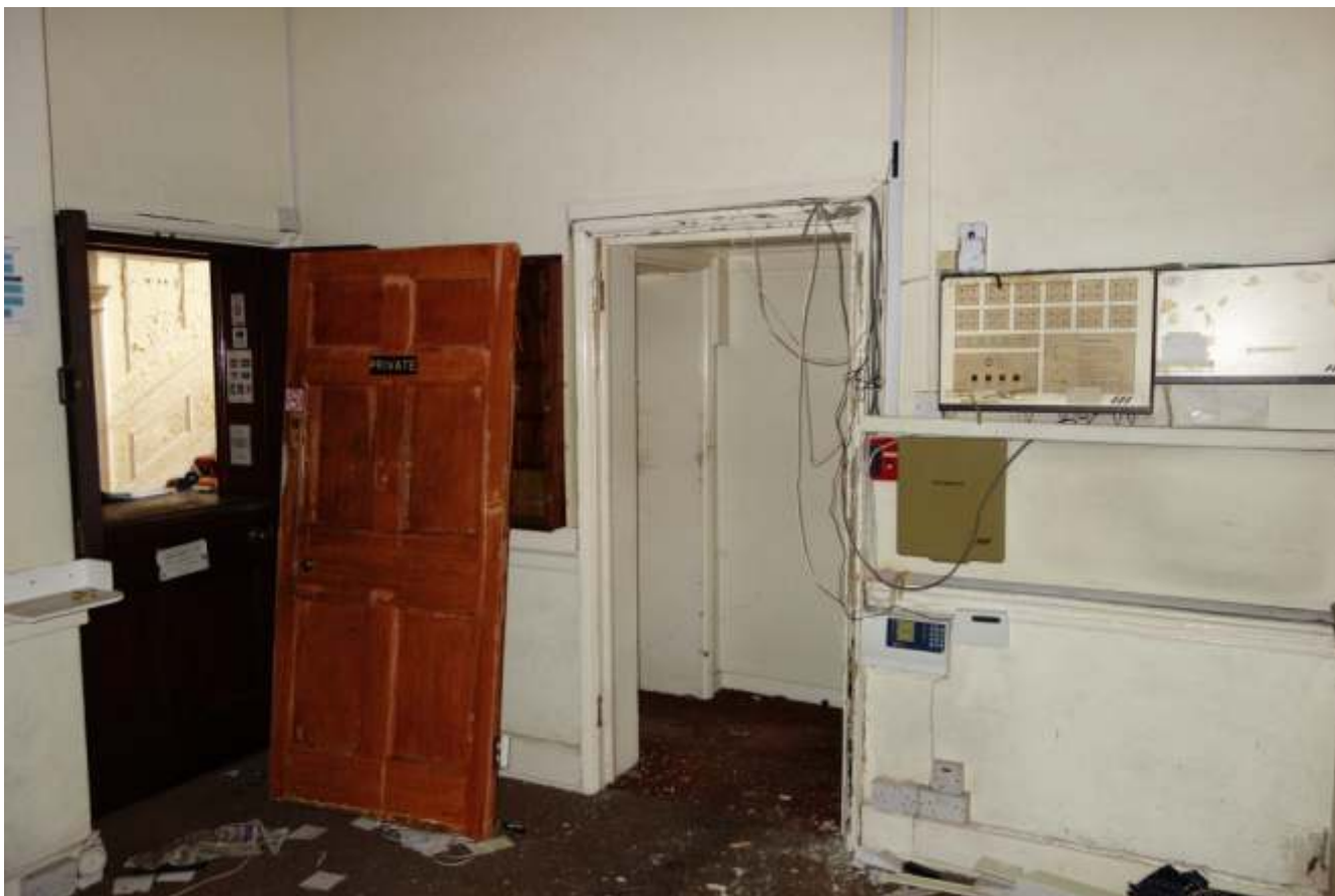
4.40: Ground floor room to north of entrance hall
