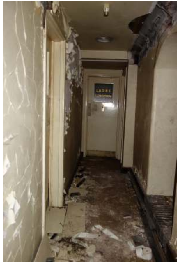
4.28: Lower ground floor corridor
