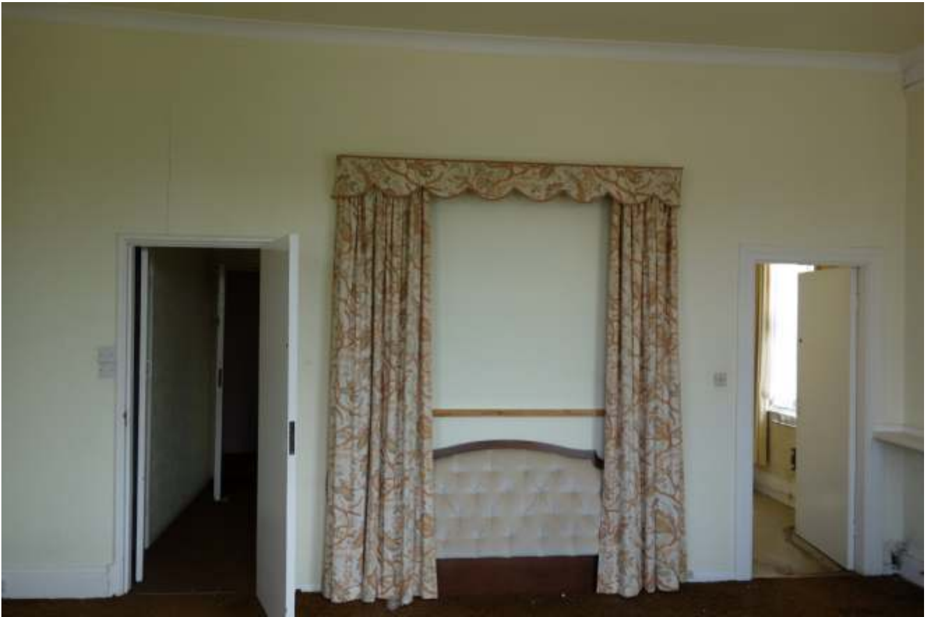
4.52: First floor bedroom: inserted partitions, corridor and en-suite within former bedroom
