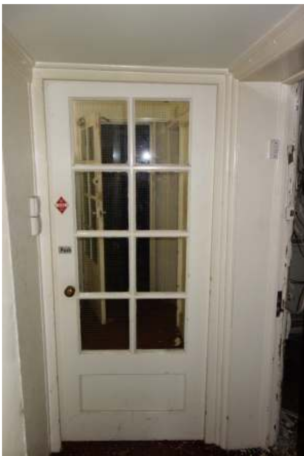
4.41: Door to north of ground floor entrance hall
