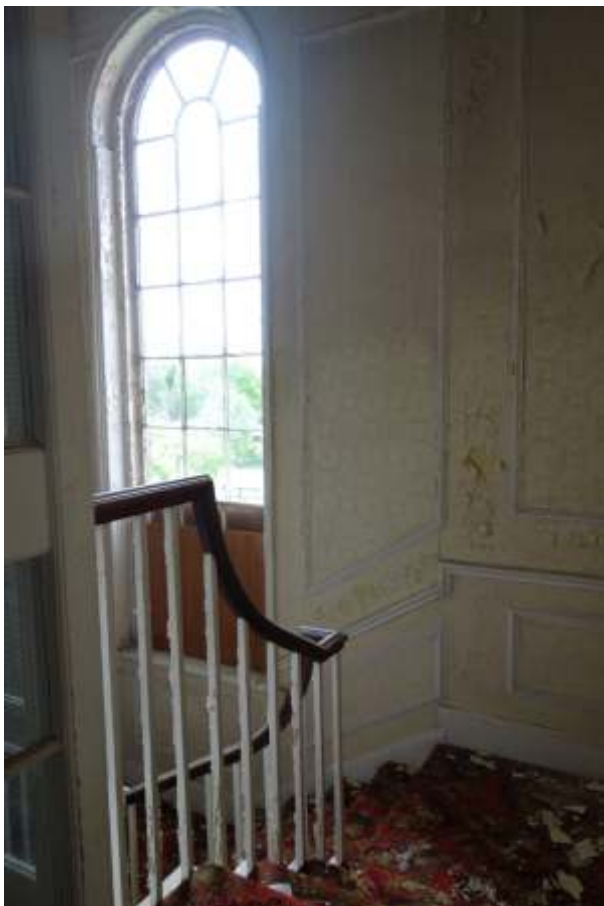
4.50: First floor landing to principal stairs
