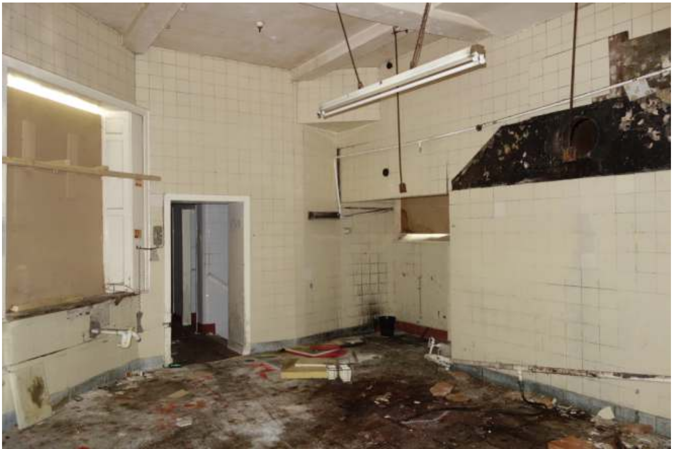
4.37: Back ground floor room converted to kitchen
