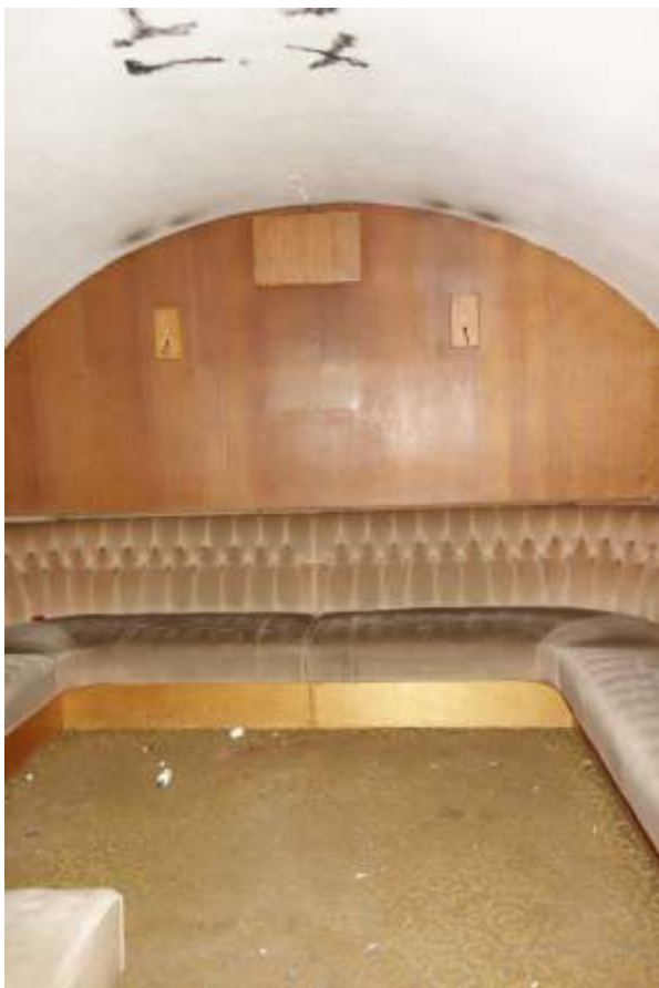
4.30: Lower ground floor typical vault to front
