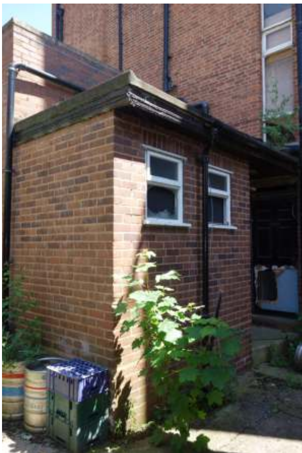
4.11: Rear wall of coach house
