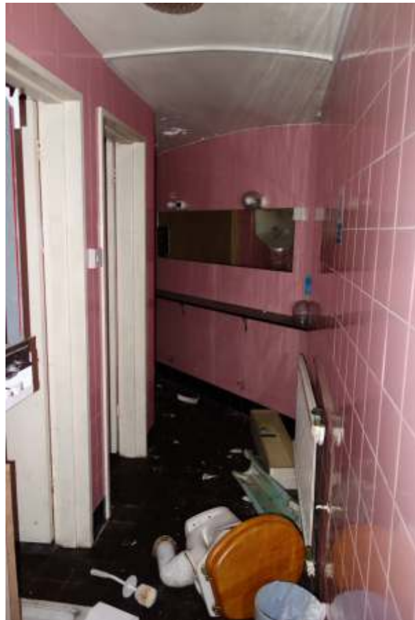
4.36: Partitioned vault at lower ground floor converted to WC
