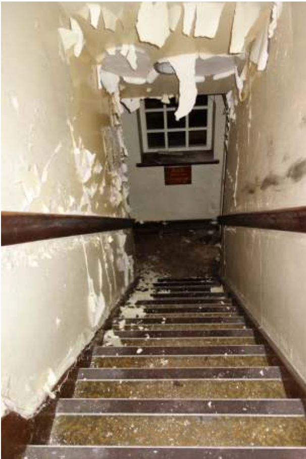
4.27: Stairs to lower ground floor
