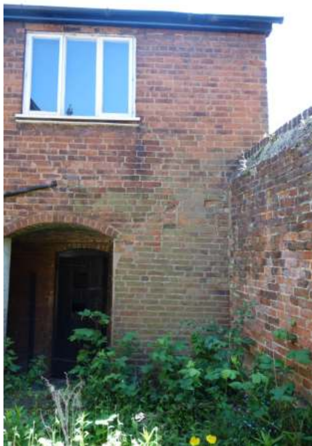
4.14: Rear wall of back range
