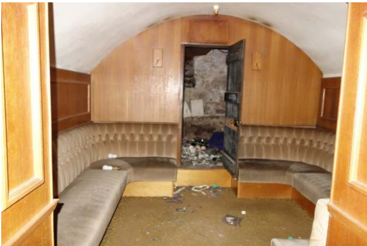
4.32: Lower ground floor vault
