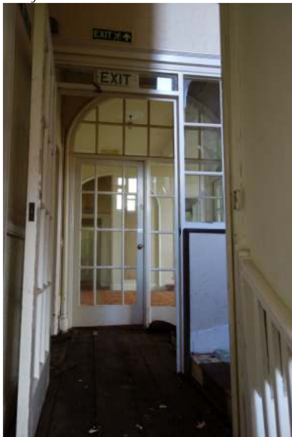
4.47: First floor landing to secondary stairs
