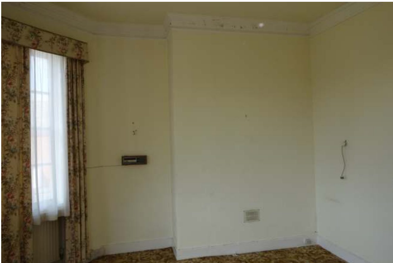
4.59: First floor bedroom to rear, north side
