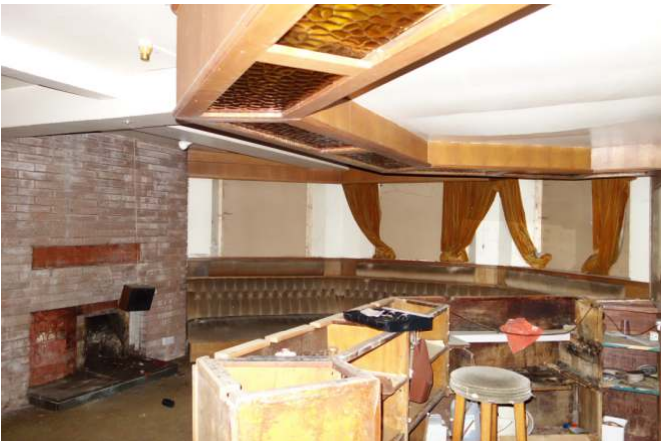
4.29: Lower ground floor back room
