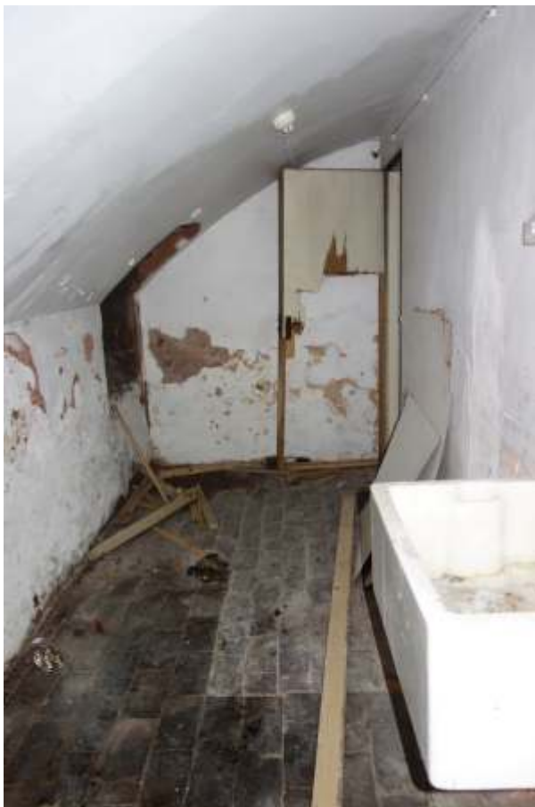
4.35: Partitioned vault at lower ground floor
