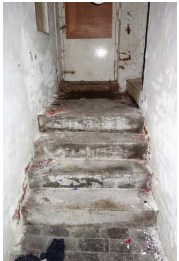
4.39: Back range stairs
