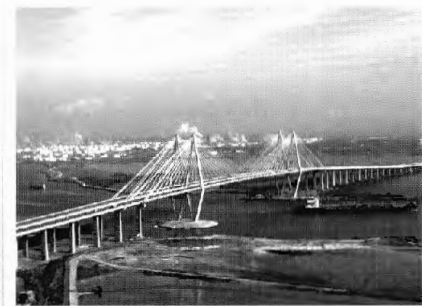
Houston's Ship Channel Bridge
