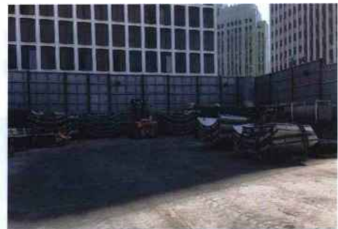
Staging Tunnel Segments at Western Yard
