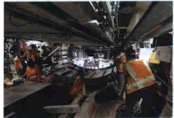
Installing Steel Rings – Purple TBM
