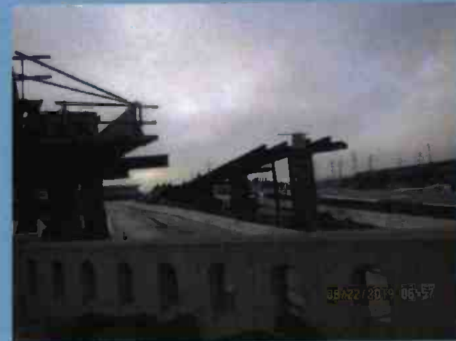
Falsework construction of Pedestrian Bridge Bent cap 2
