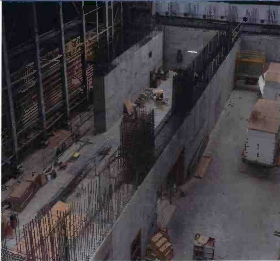
Interior wall progress overview
