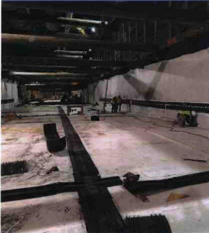
HDPE installation at south Flower St
