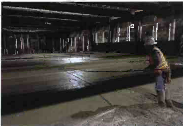
Mud Mat Placement
