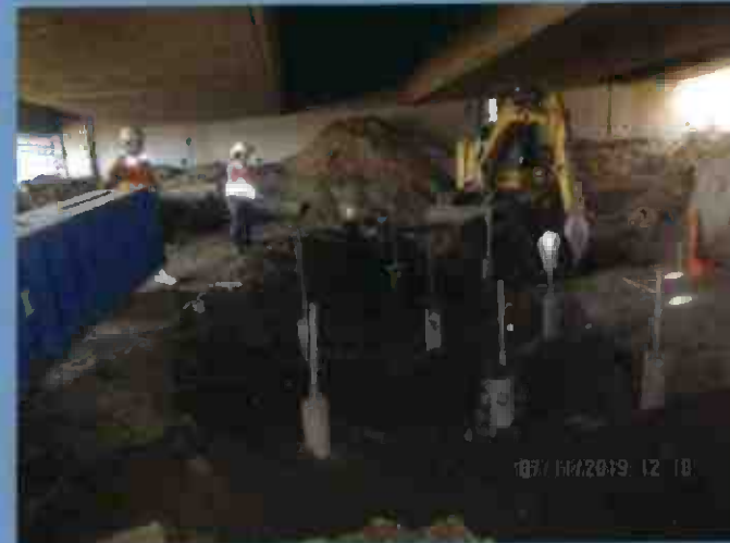
Ped Bridge Bent 1, 2, and 3 micropile installation
