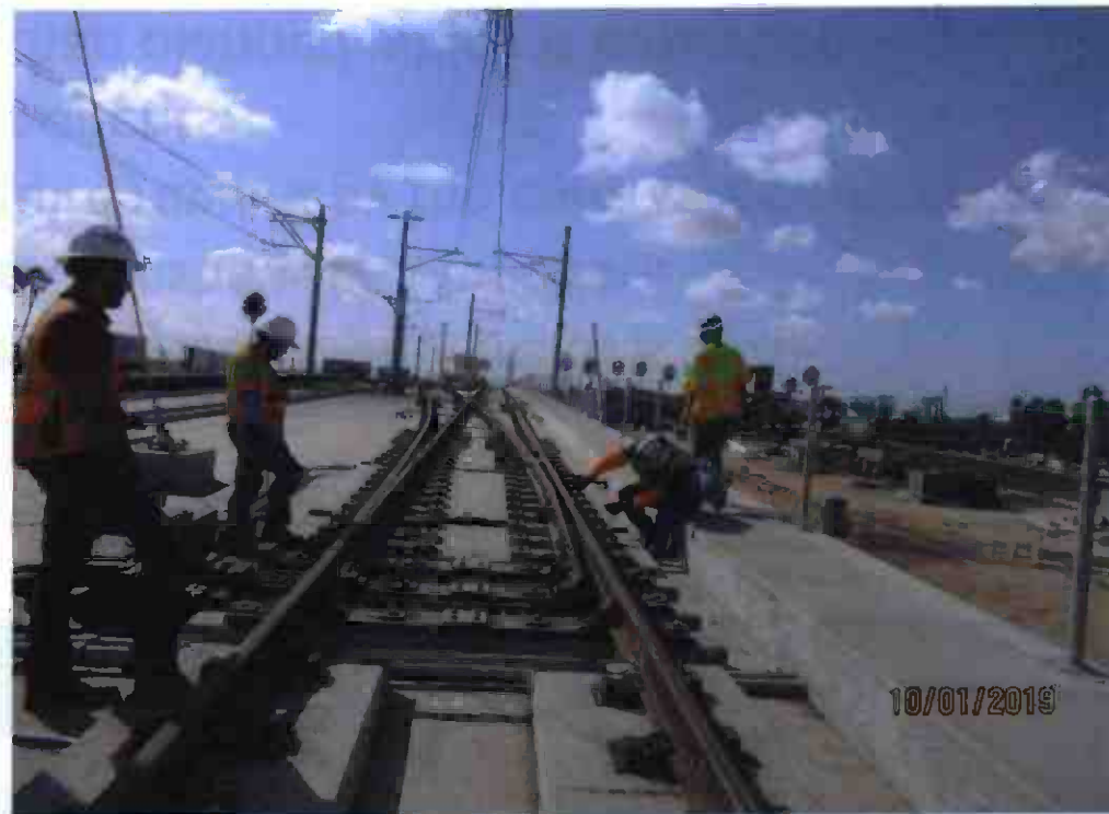
Century Bridge – Inspectors on SB Track measuring TOR
