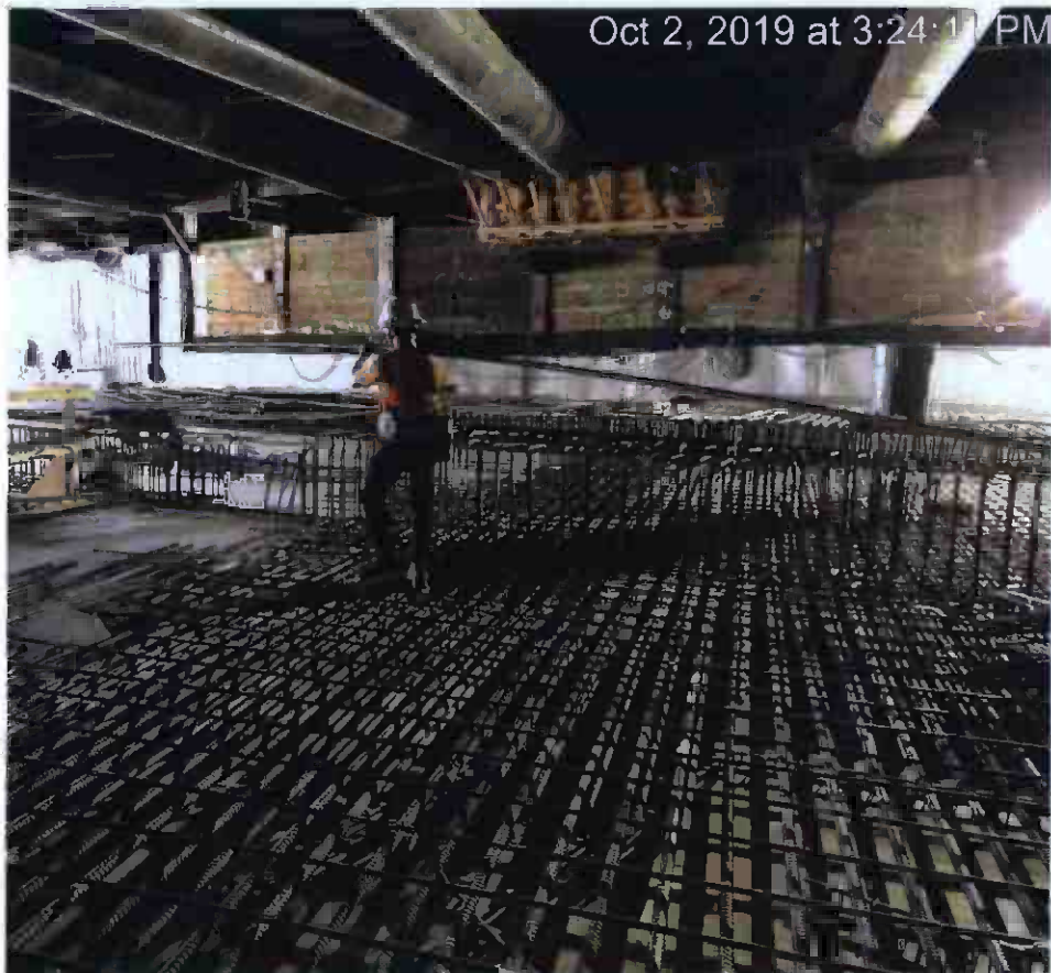
Bottom mat rebar installation for track roof slab
