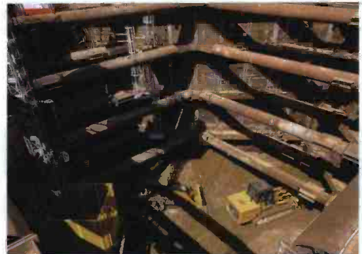
Tunnel Access Shaft Excavation
