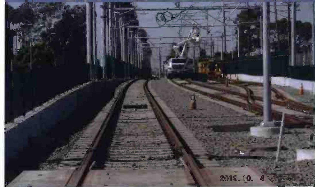
High Street – OCS work siding track area
