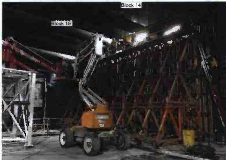
First Lift Wall Concrete Placement
