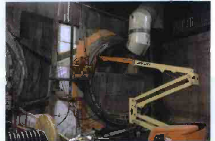
HDPE Installation at East Bulkhead
