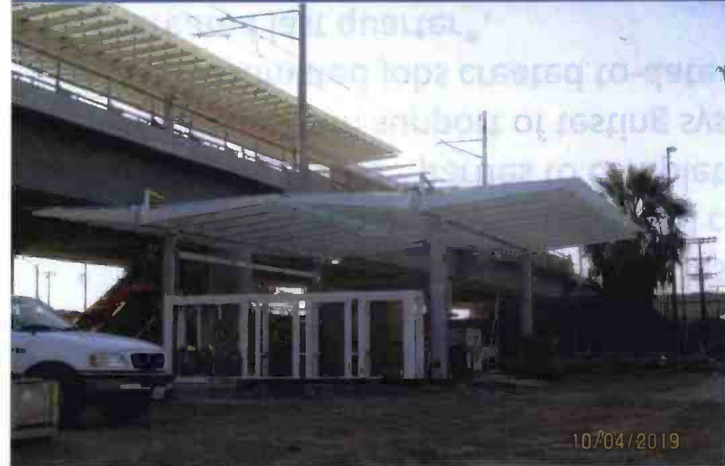
Aviation Station – Glass panel installation at ticket kiosk
