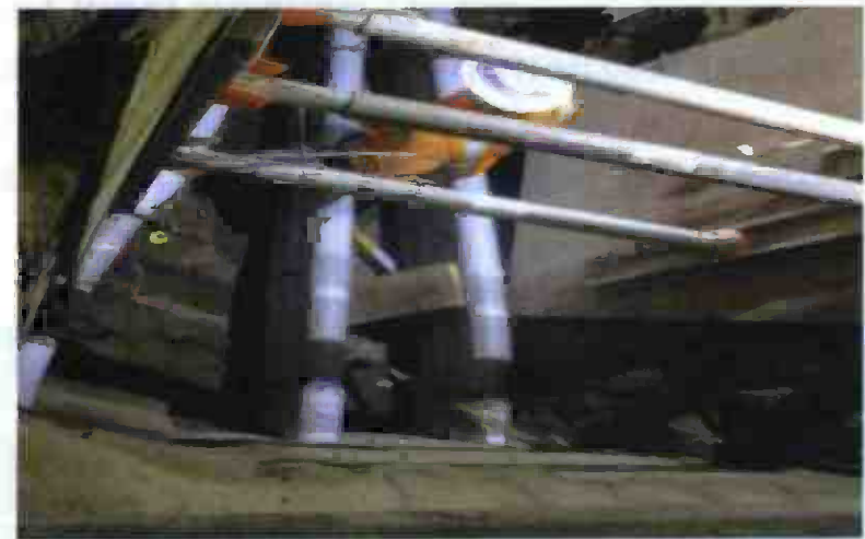
Telecom Main Line A and Lateral A6 Installation
