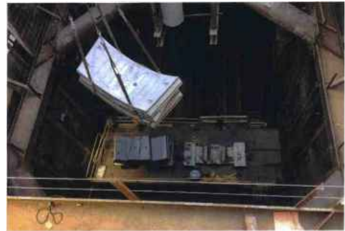
Lowering Tunnel Segments at Western Yard
