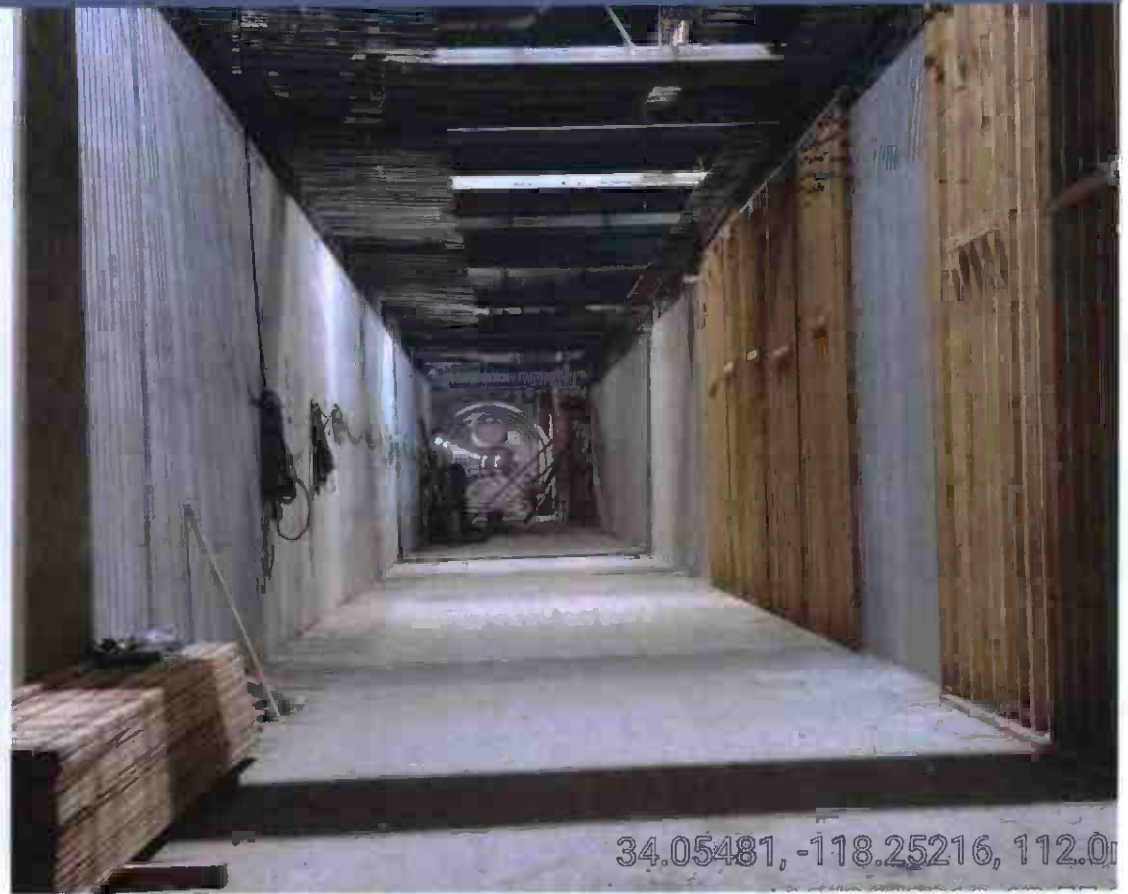
Left Track Tunnel at Flower St
