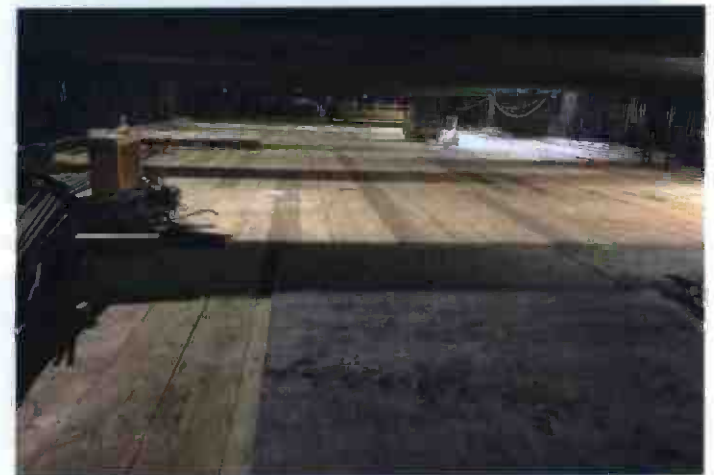
Decking at High Bay Platform
