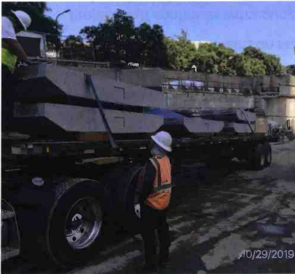
Floating Slabs delivery at Grand Av Arts/Bunker Hill Station
