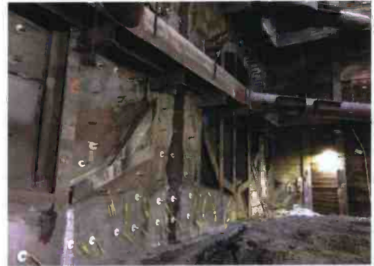
TBM Launch Box Excavation
