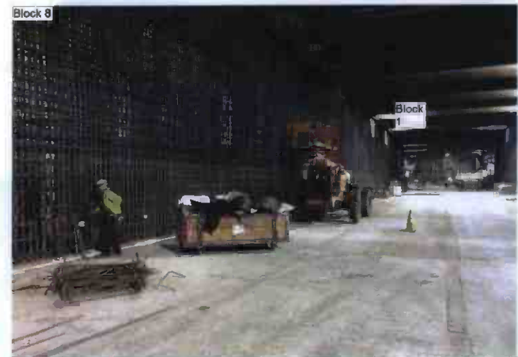
Wall Rebar Installation
