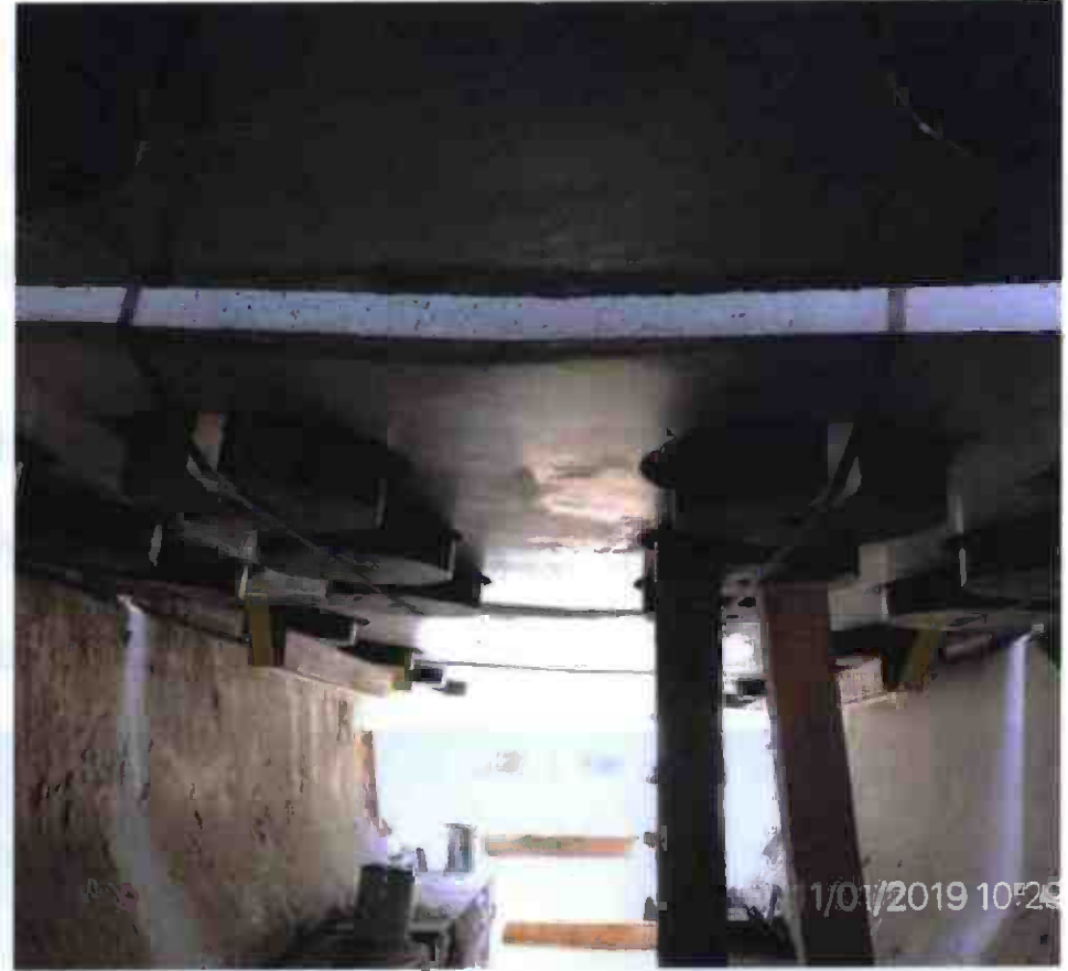
Gluing of bearing pads to Floating Slabs 4
