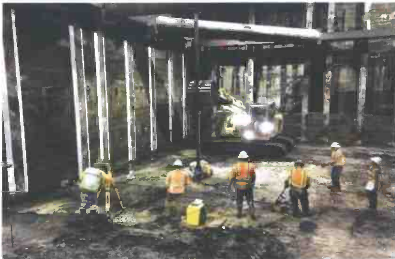
Wilshire/Fairfax Station Geotech Testing
