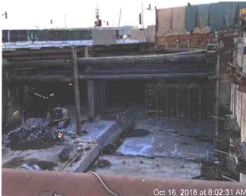
Oct 16, 2018 at 8:02:31 AM Installation of mud slab at track level
