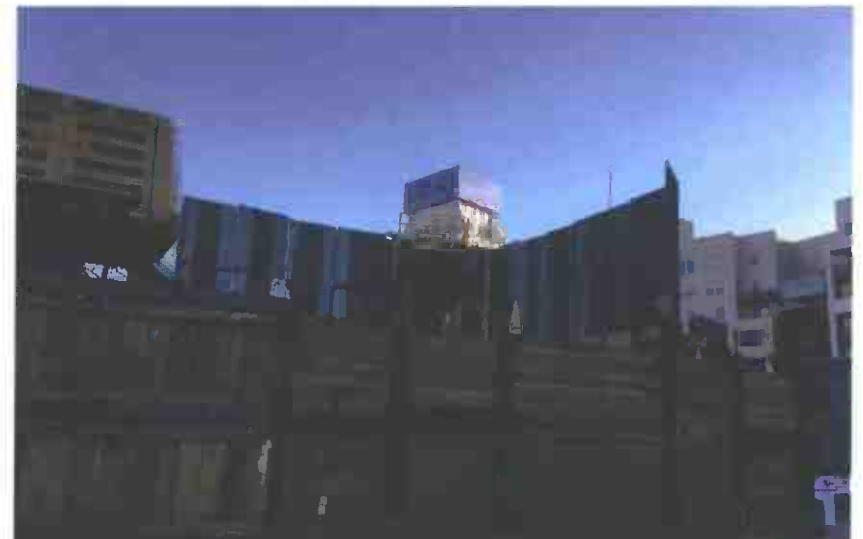
View of South Yard Muck Pit at Wilshire/La Brea
