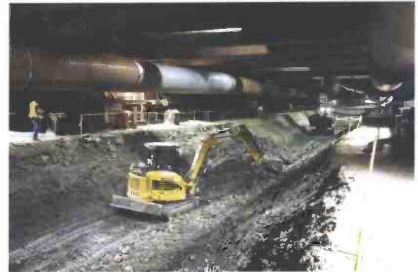
Wilshire/La Cienega Station Excavation
