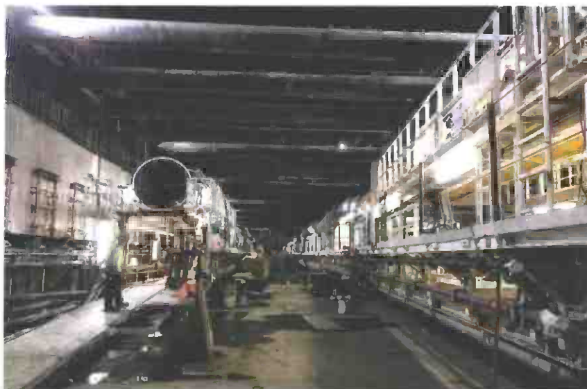
View of Both TBMs – Looking East
