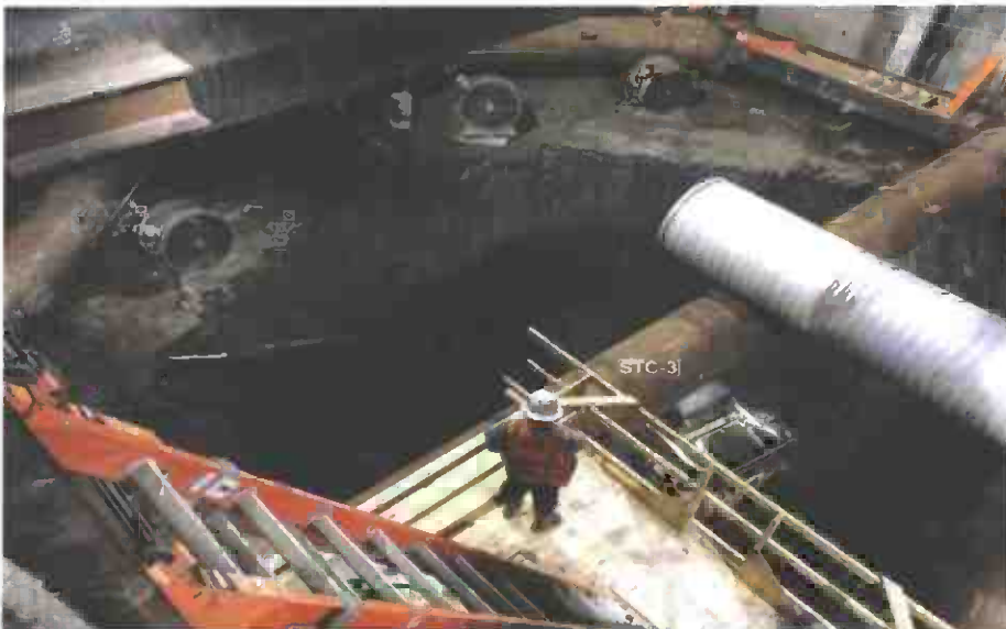
Wilshire/Western Excavation below Level C
