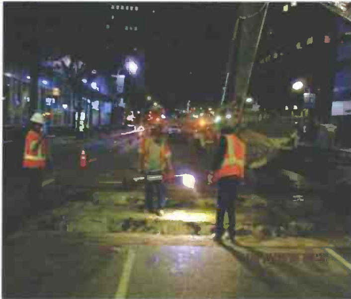
SBCC placing backfill over Ex-Vent at Gayley and Wilshire
