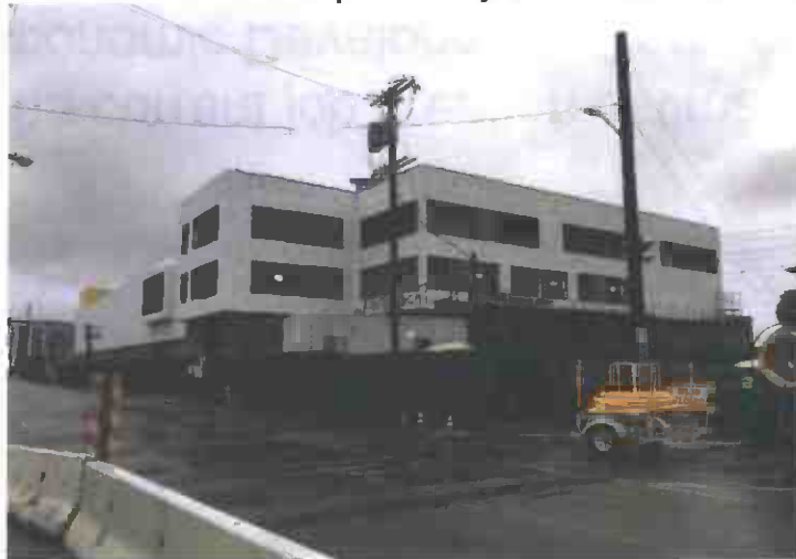
Division 20 MOW Building – View Looking North-East
