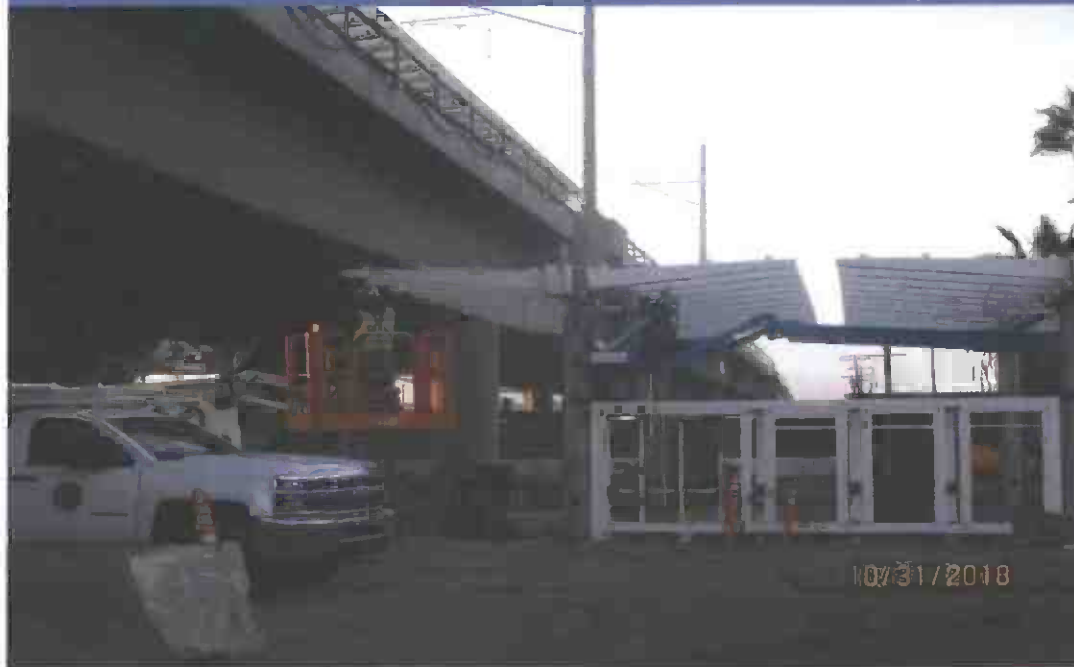
Rain gutter installation for the Aviation/Century Station ticket kiosk canopy
