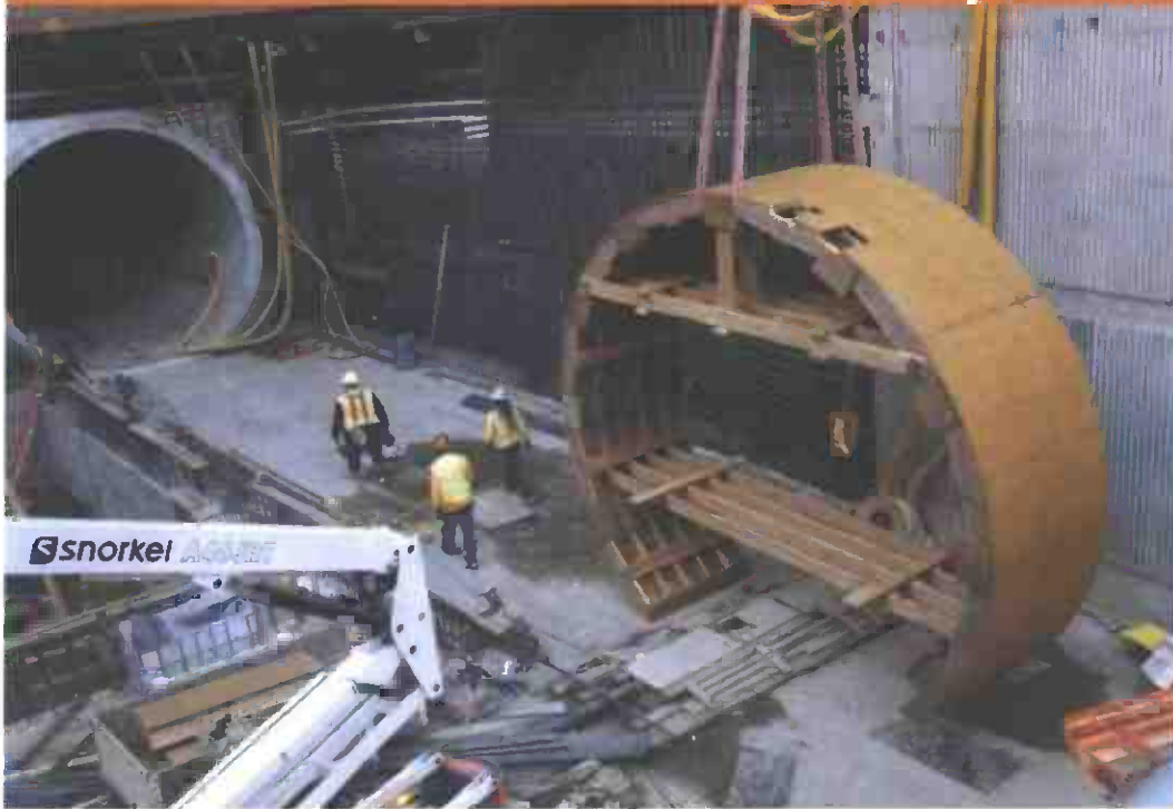
Tunnel Eye formwork at East Hammerhead
