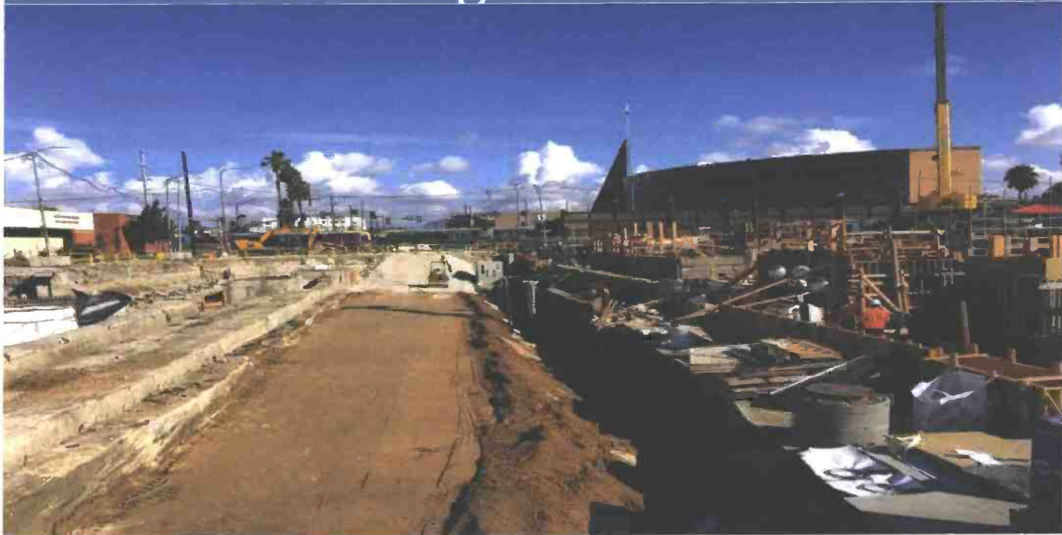
Crenshaw Blvd. restoration and Expo/Crenshaw Station entrance construction near Expo Line.
