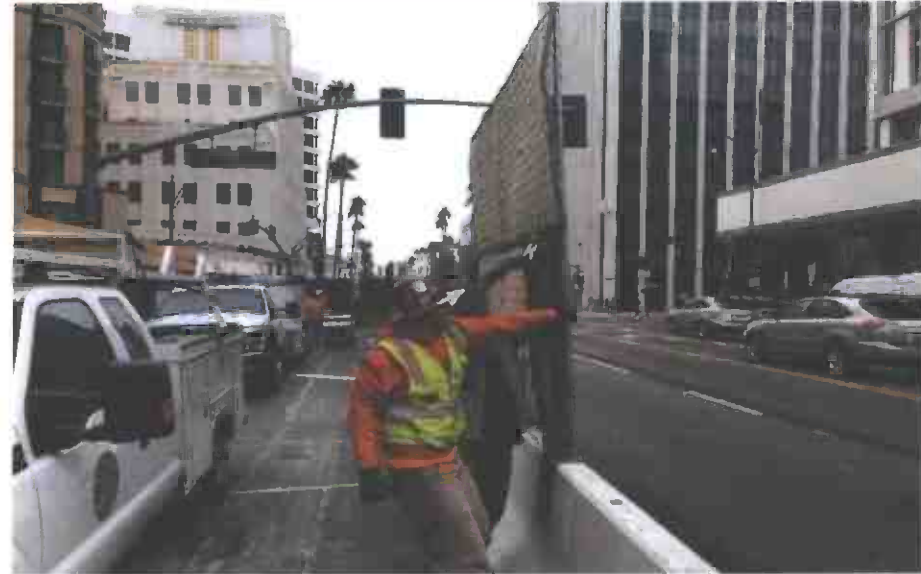
K-Rail Installation in Beverly Hills
