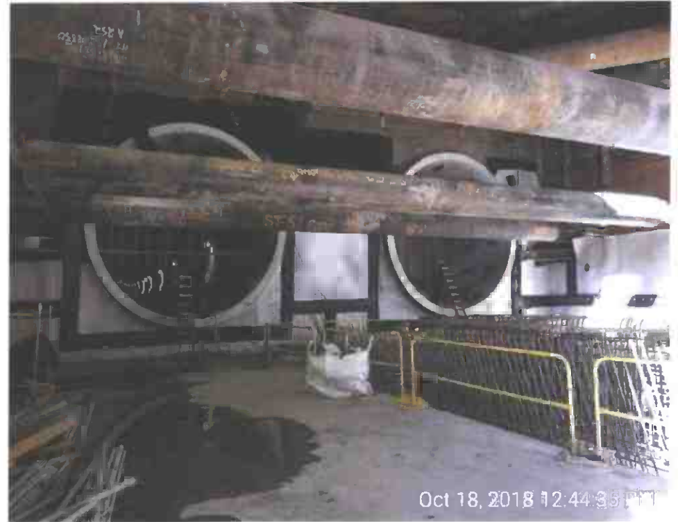
HDPE installation around tunnel eyes
