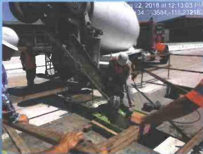
Pouring Bent 6C for the emergency stairway exit
