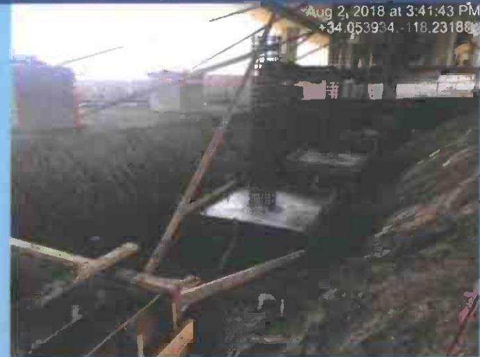
Poured column footing at emergency stairway exit
