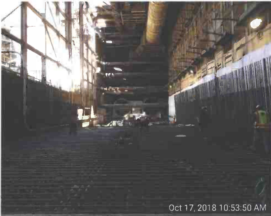
Rebar installation of top mat
