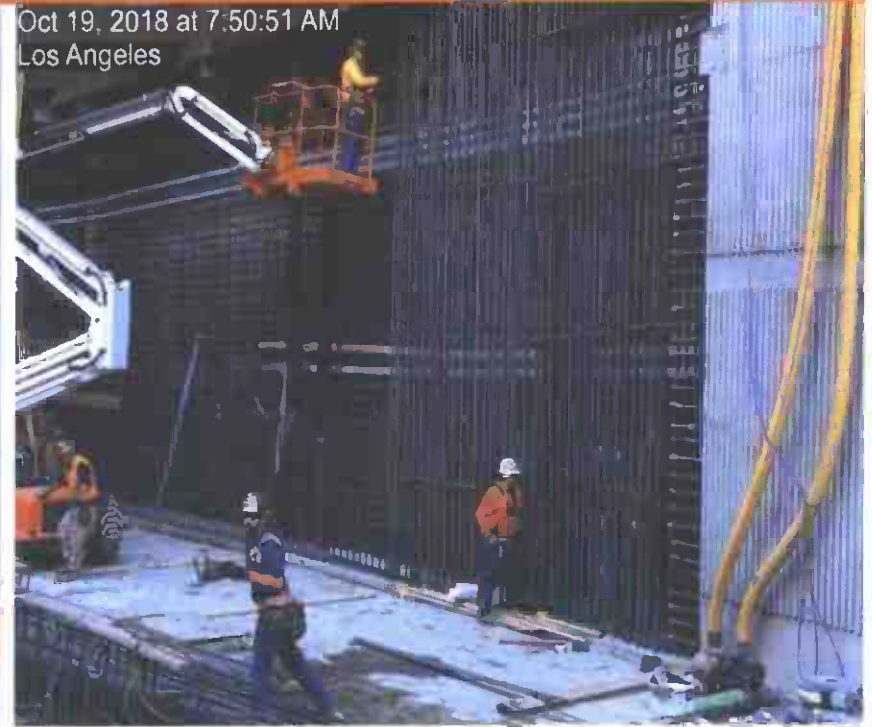
MEP installation at East Hammerhead
