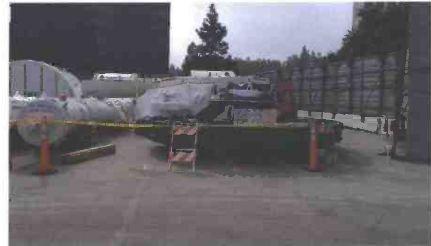
TBM Delivery in Century City
