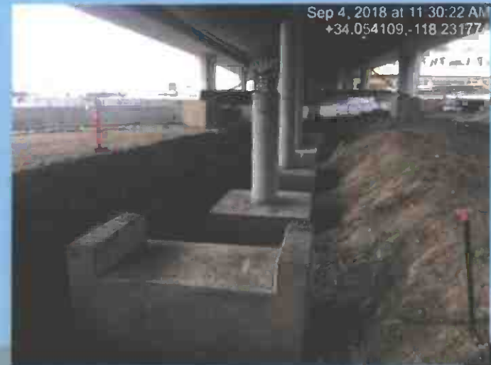
Cured Bents 6C-9C for the emergency stairway exit
