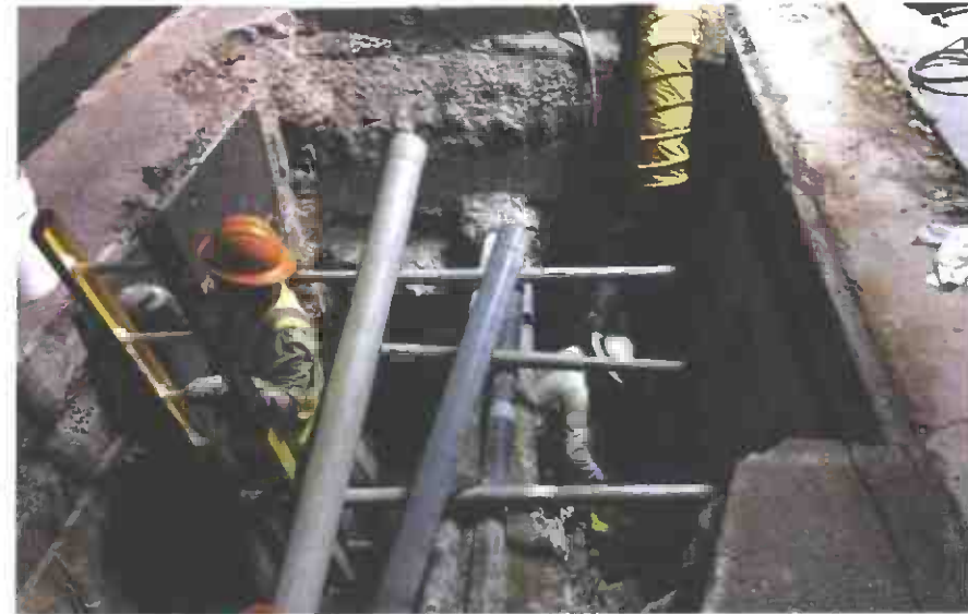
DWP Power Conduit Work in Century City
