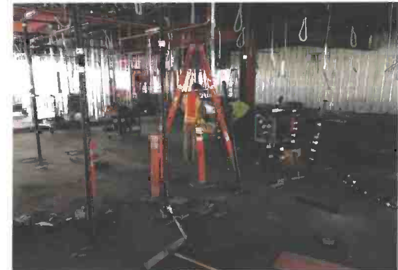
Division 20 MOW Building – 1 st Flr Maintenance Bay
