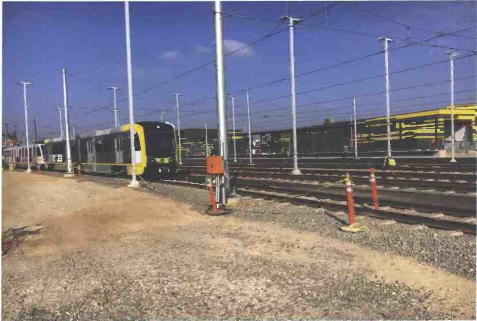
Southwestern Yard – Four LRT Vehicles moved into yard for support of systems testing
