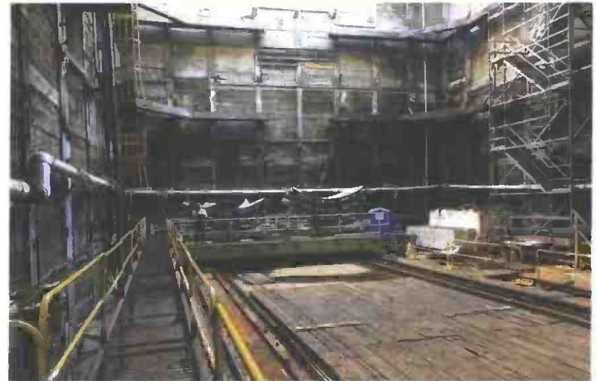
Tunnel Segments on Car Passer at Wilshire/La Brea
