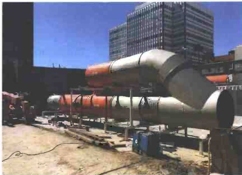
Fabricating Ventilation Ducts at Wilshire/La Cienega Station
