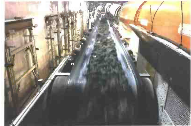
Wilshire/La Brea Station – Muck on TBM Belt Ring
