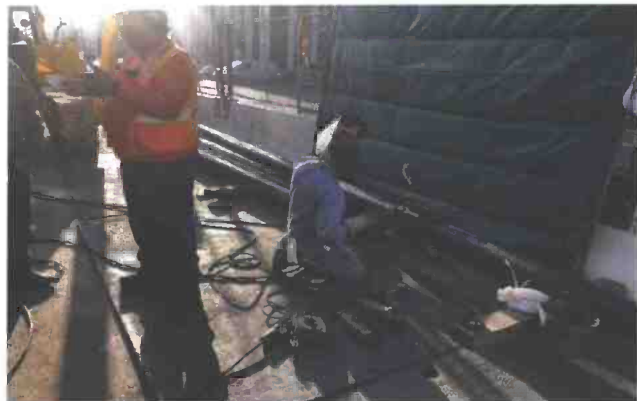
SCG Welding Pipe in Beverly Hills
