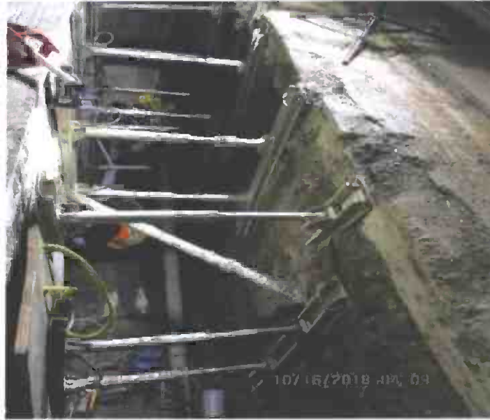
Conduit Placement at Gayley and Wilshire
