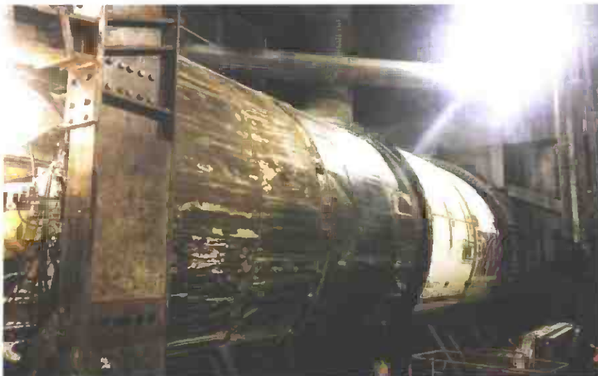
Launching TBM at Wilshire/La Brea Station
