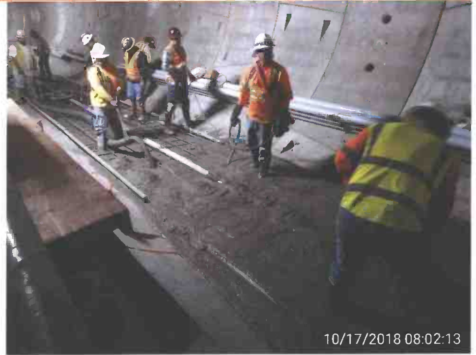
Concrete placement of Left Tunnel Invert, Hope to Broadway
