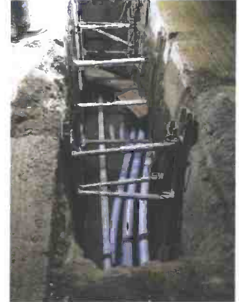
Conduit Placement at Gayley and Wilshire
