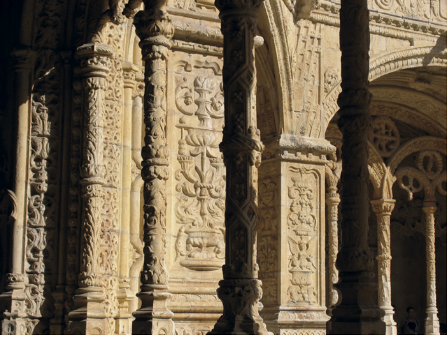
FIGURE 5.3 Detail of the cloister of the monastery of Jerónimos, Lisbon IMAGE © NUNO SENOS
