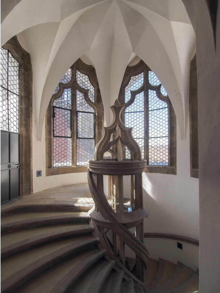
FIGURE 19.2 Arnold of Westfalen, Albrechtsburg in Meißen, Great Staircase Tower (ca. 1485) IMAGE © AUTHOR
