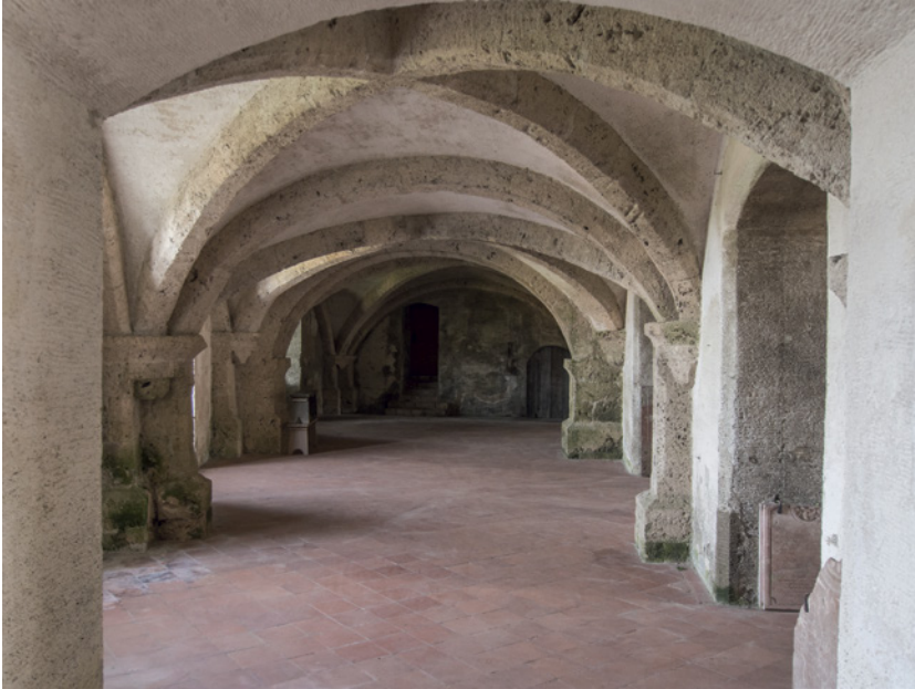
FIGURE 19.6 Ulrich Pesitzer (attributed), Burghausen (Bavaria), ground floor hall with a Romanesque Renaissance vault (ca. 1480)
