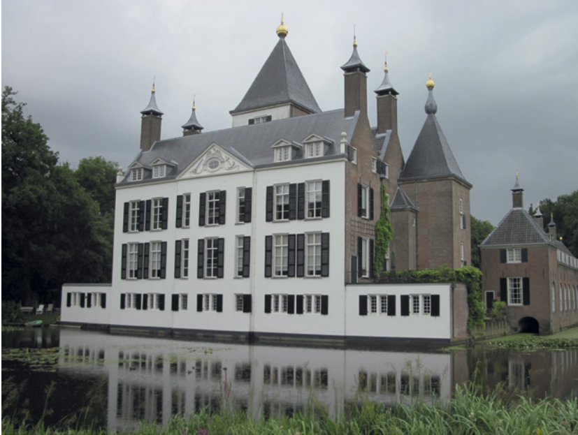
FIGURE 12.12C Renswoude Castle, rear facade, plastered in the early 19th century IMAGE © STEPHAN HOPPE
