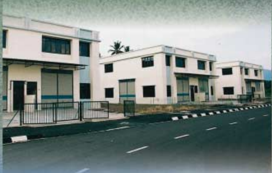
Permatang Tinggi Double Storey Semi-Detached Light Industry Factory
