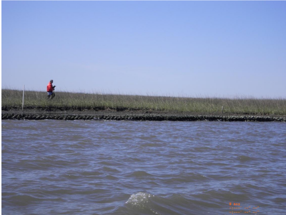
Photo 3: View of Reach A A-Jacks looking west
