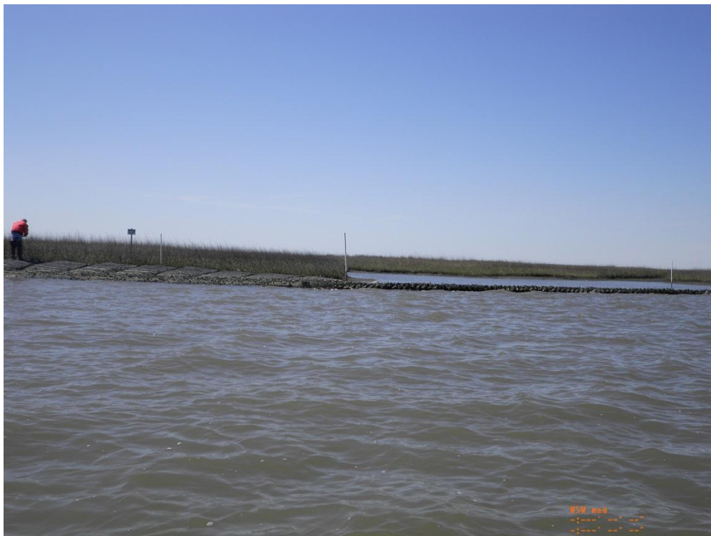
Photo 6: Transition between Gation Mats and A-Jacks on Reach B
