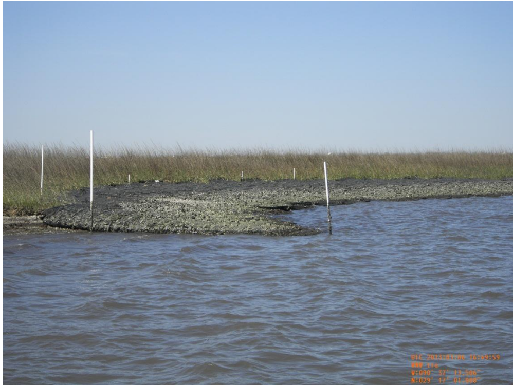
Photo 1: Gabion Mats located on the southern end of Reach A looking north
