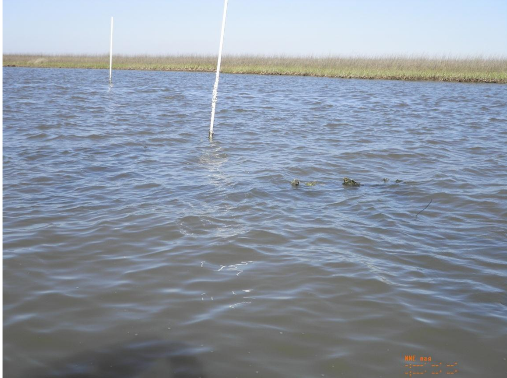
Photo 15: Transition from Gabion Mats to ReefBlks on Reach E submerged
