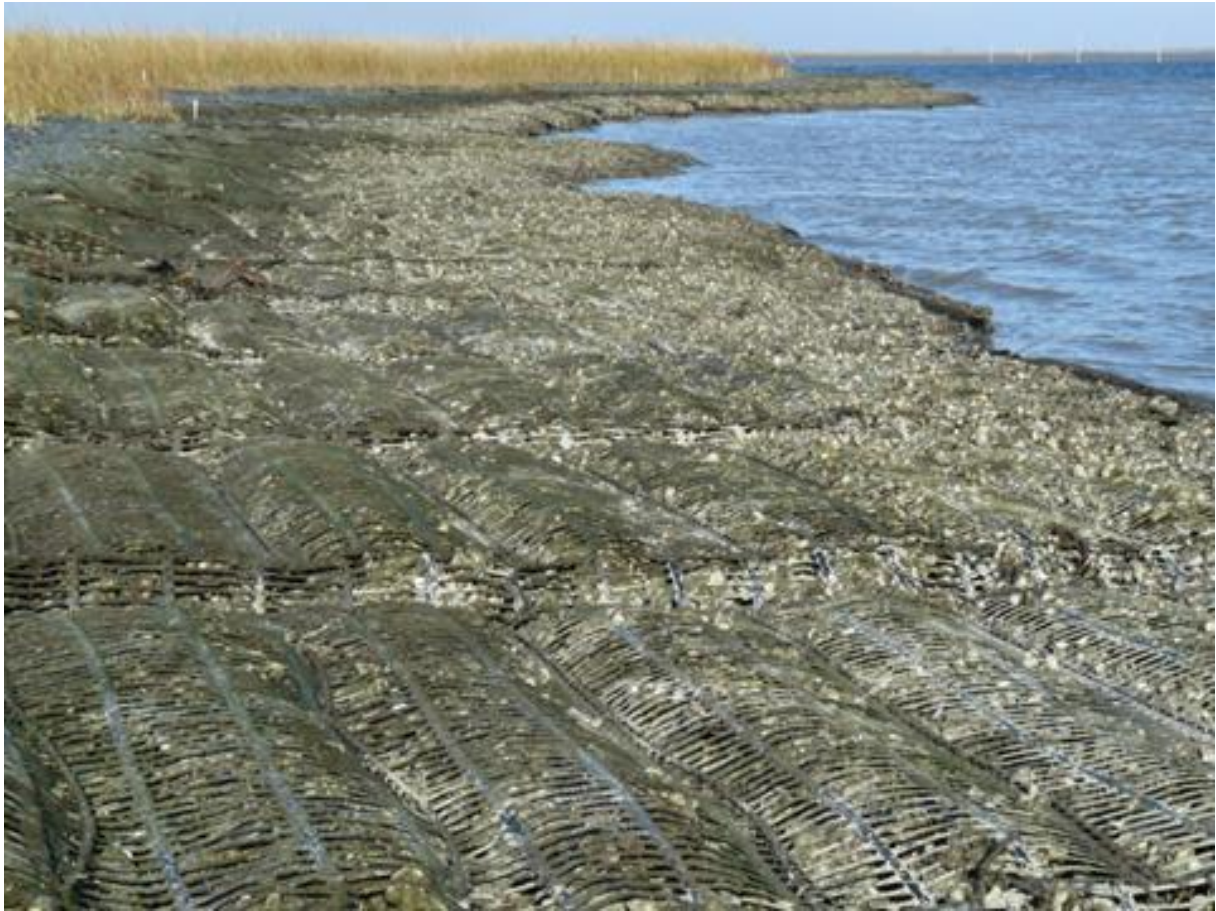
Figure 24. Reach A Gabion Mats showing oyster population gradient from top of mat (to the left in the photo) to the bottom edge of the mat. Photo taken at extreme low tide in winter.
