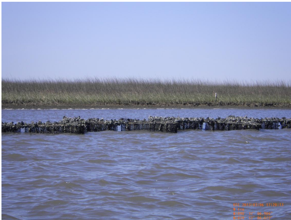
Photo 4: View of Reach A ReefBlks looking west
