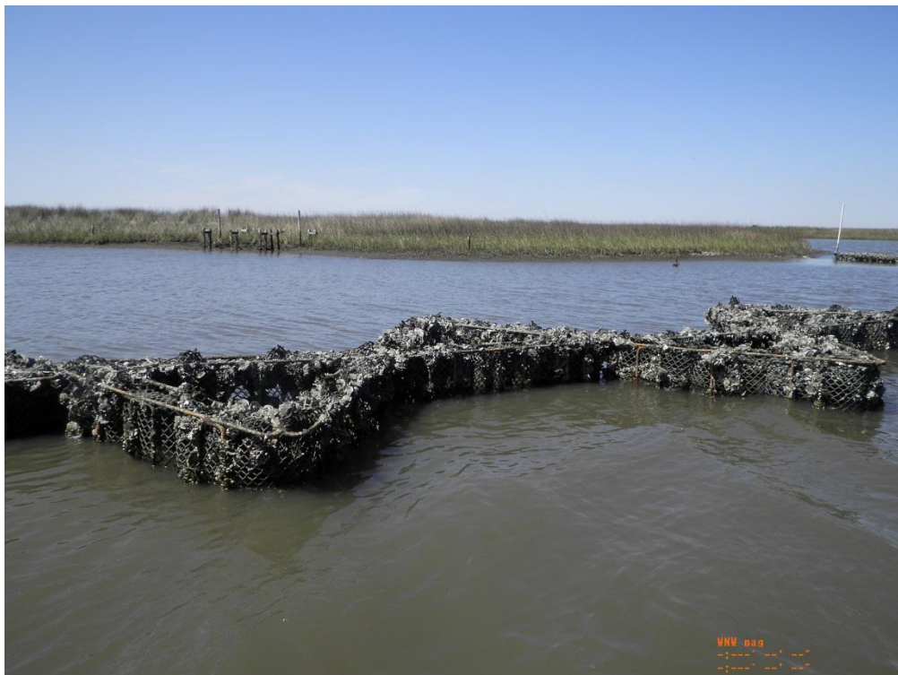
Photo 8: Close up view of ReefBlks on Reach B
