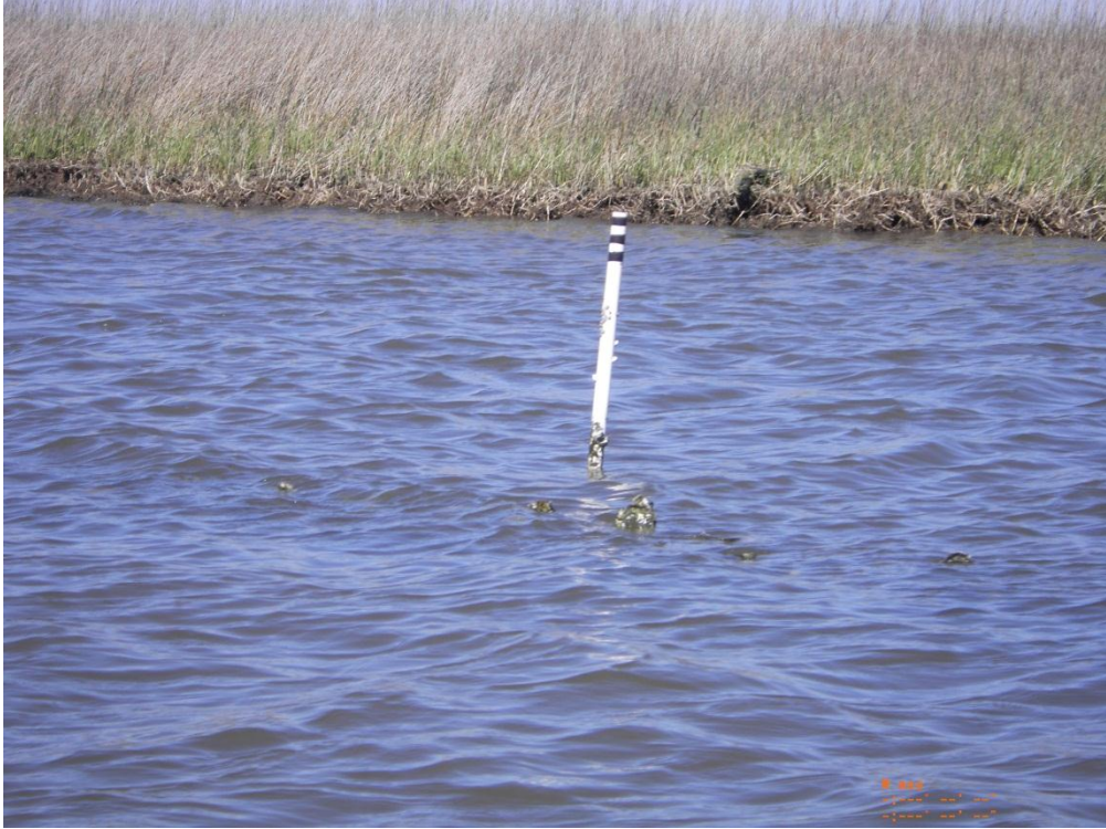
Photo 17: View of submerged A-Jacks on Reach E
