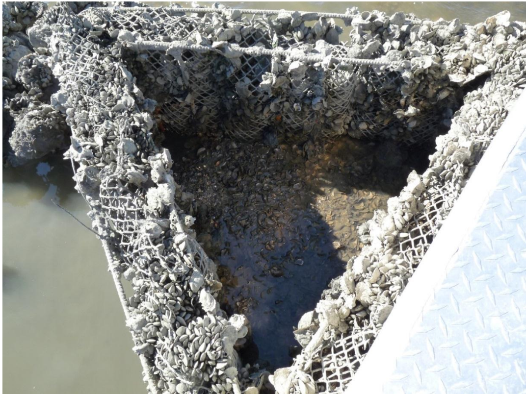
Figure 46. Photo showing oyster shell and mussel shell deposition with the ReefBlk triangle during the winter 2011-12 assessment.
