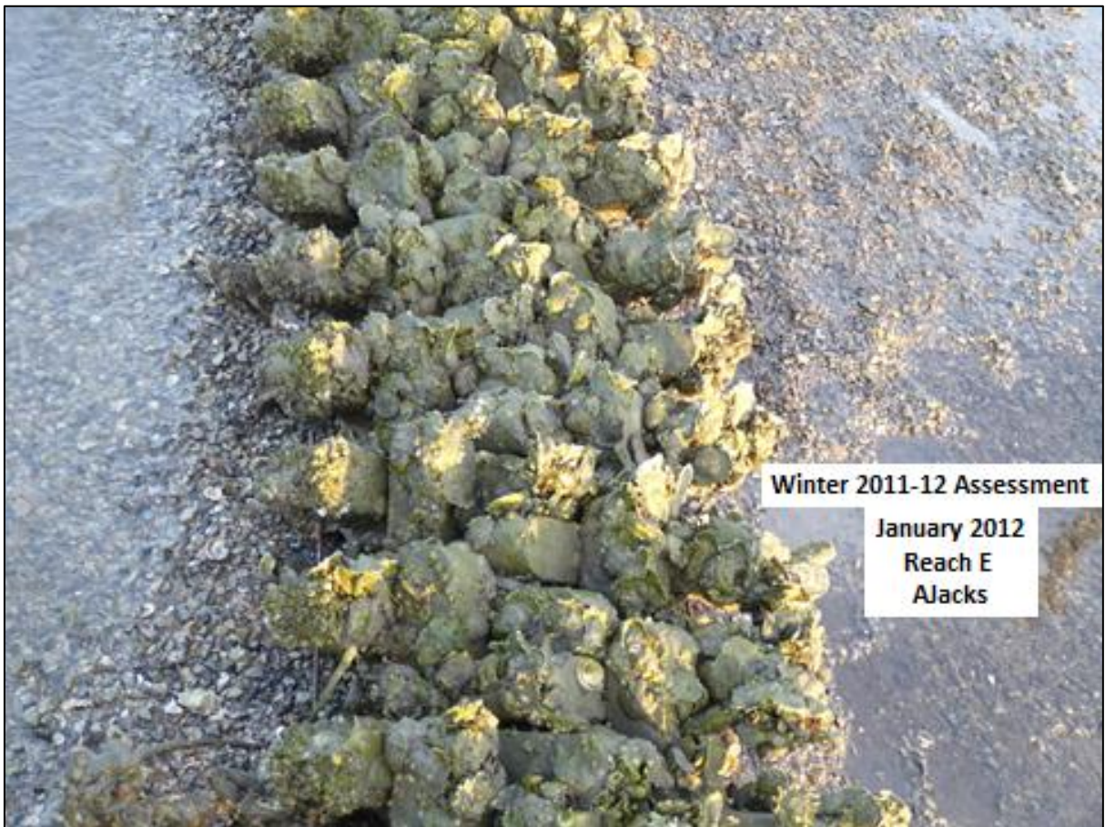
Figure 35. Photo of A-Jacks showing surficial oyster coverage and oyster reef development as well as bare areas during winter 2011-12 assessment.
