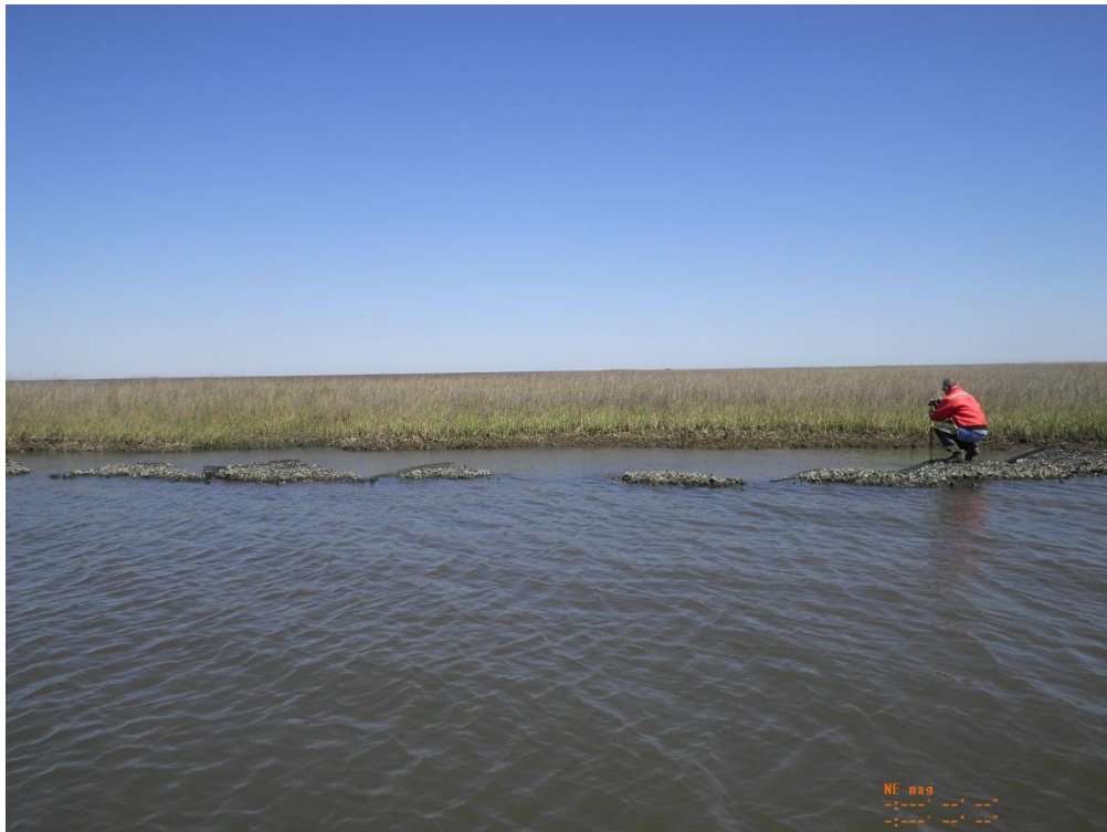
Photo 14: View of Gabion Mats low area on Reach E looking east
