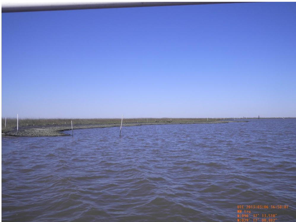
Photo 2: Gabion Mats located on the southern end of Reach A looking north
