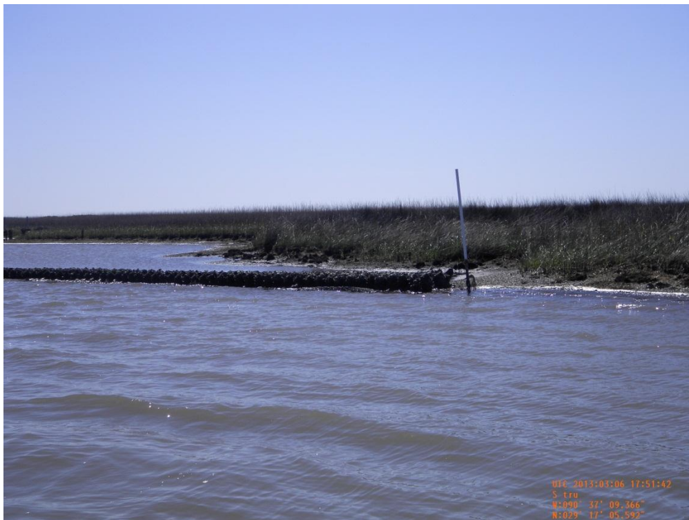
Photo 10: View of shoreline tie-in on north side of Reach B
