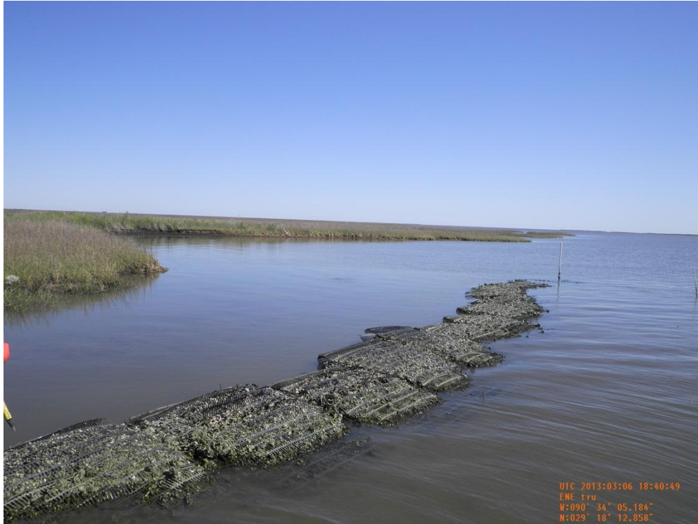
Photo 11: View of Gabion Mats on the south end of Reach E looking south
