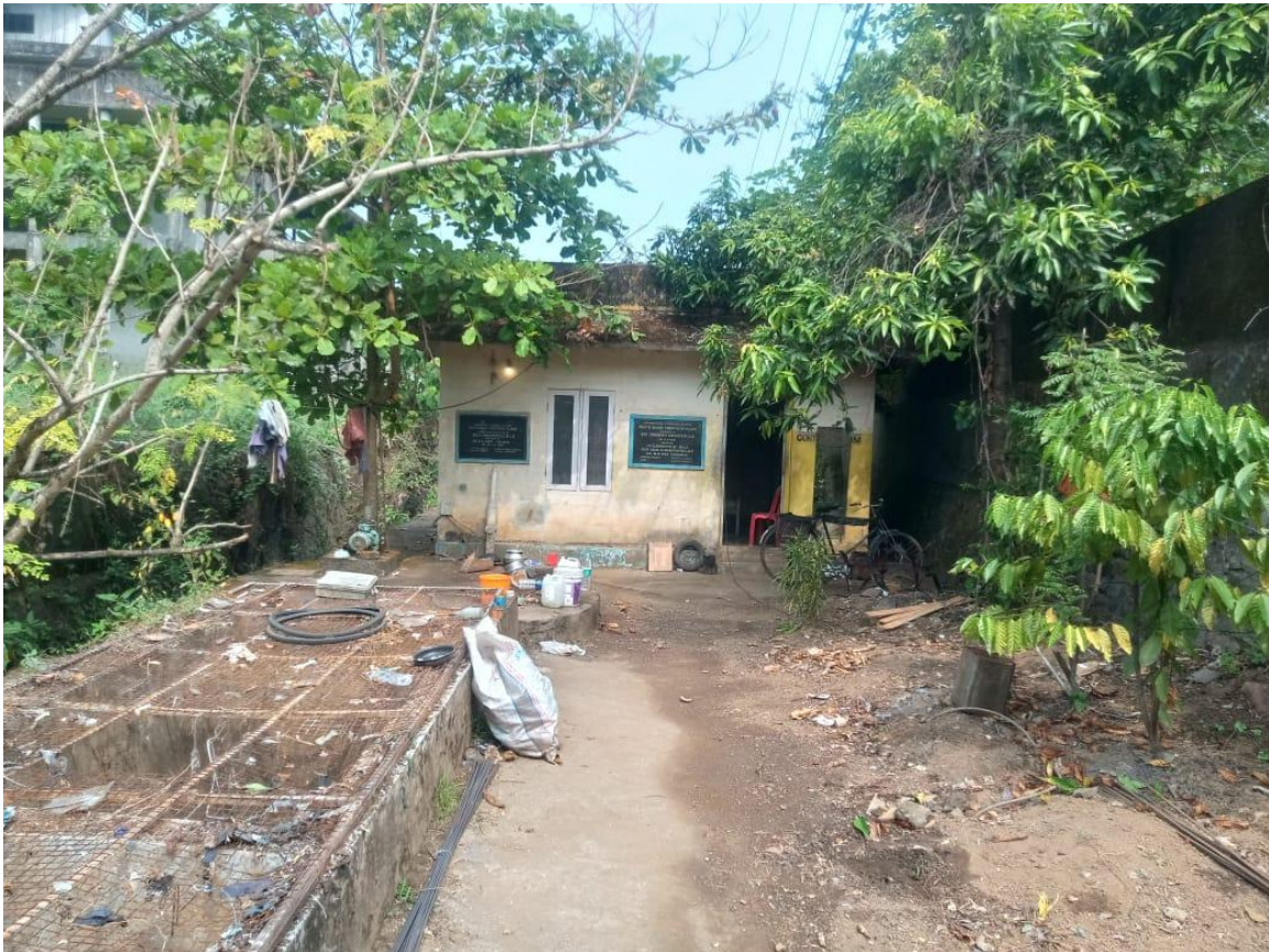
Fig.2.1 Existing Storm Water Treatment Plant at Aluva
