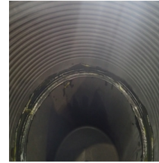
Figure 10.1.4 – O-ring fitted (Cap)
