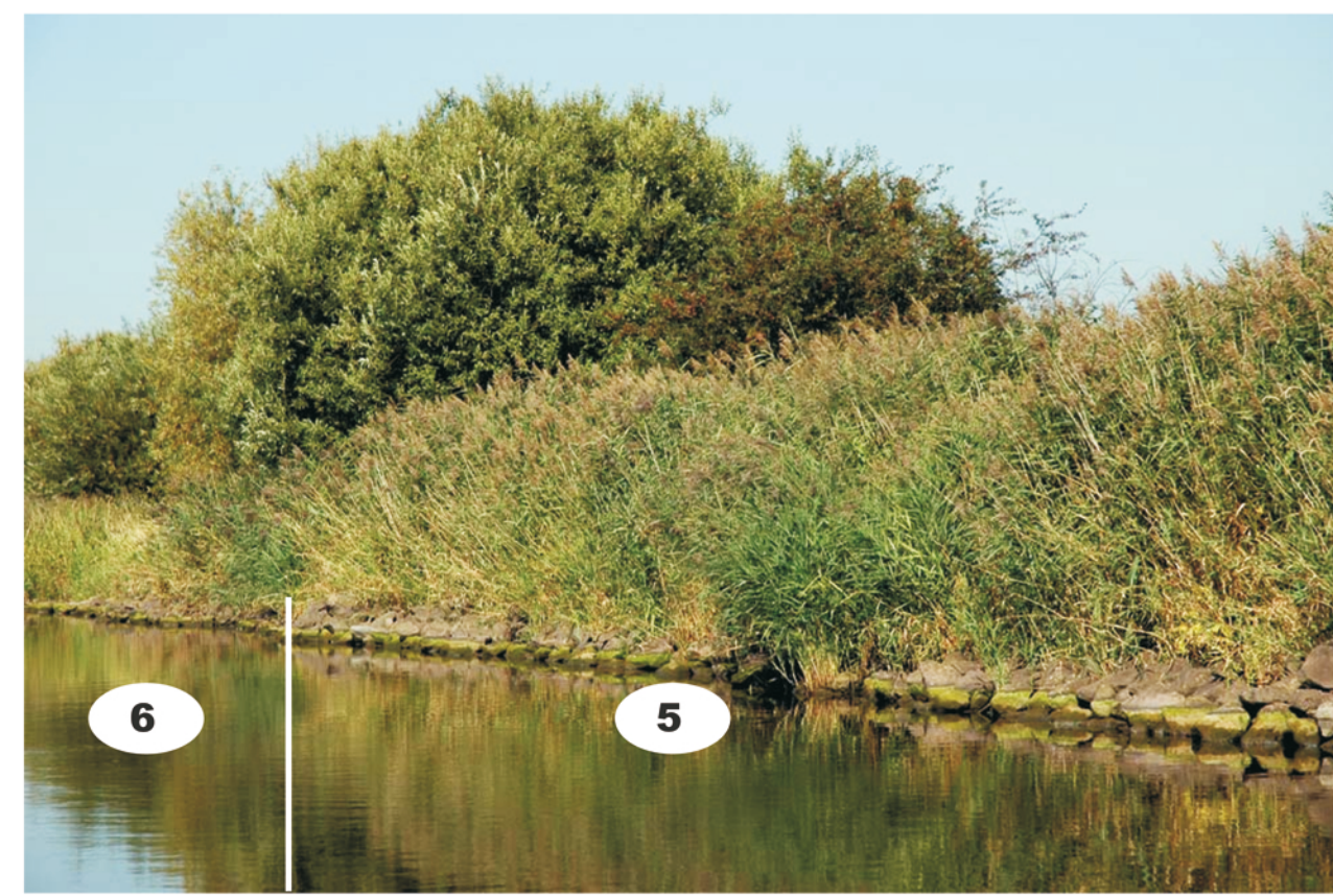
Site of photograph: groyne 3, looking downstream
