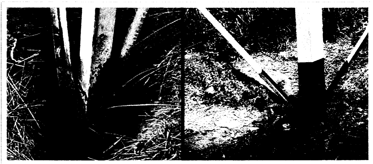
Figure 6.11.1 – Before/After Photos of a Typical Direct-Buried Steel Tower Leg
