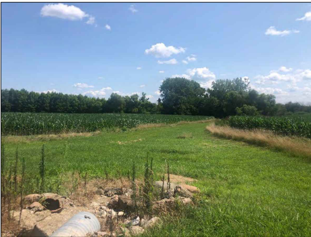
Photo 7: Photo of typical vegetated swale with road culvert on a mapped NWI headwaters. Located near the N County Road 100 E and E County Road 700 N intersection in the Project area buffer, facing south.
