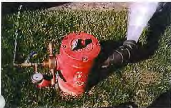
Figure 2 | Sampling device installed on the fire hydrants.
