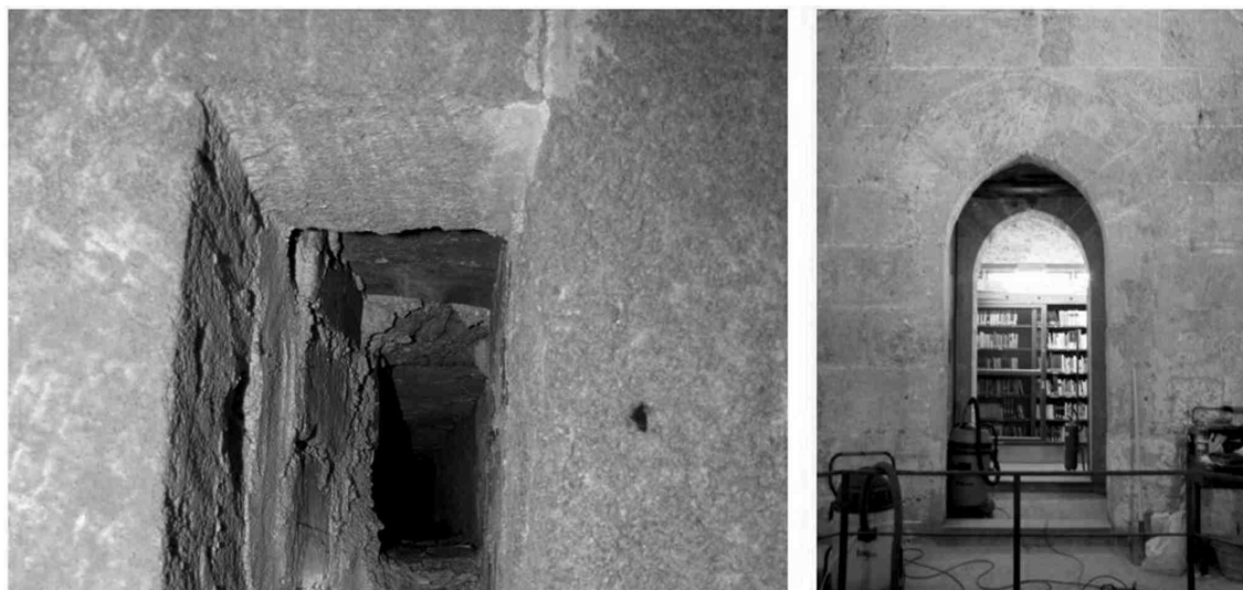
Figure 33: Left: deep hole to host the bolt locking the door of the Treasury Hall; right: the double-door inside the Treasury Hall (Photographs © Ruggero Longo).
