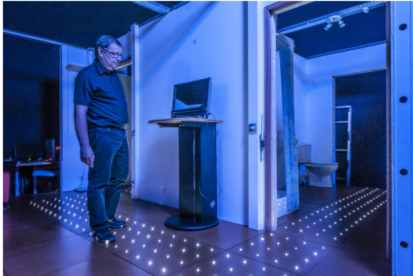
Figure 3.18 – The floor providing visual guidance to the bathroom at night
