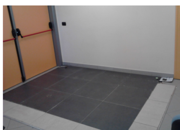
(a) The installed floor prototype
