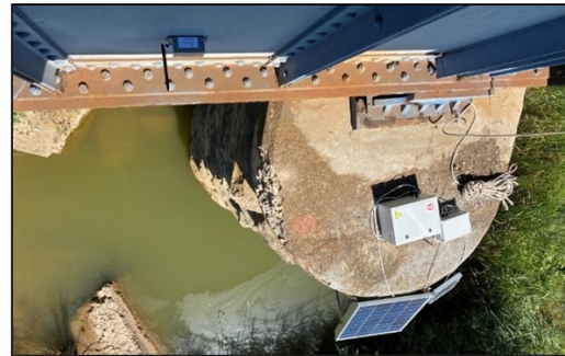
Figure 3: Hardware installed on the bridge.
