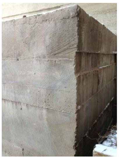
IMAGE OF FINISH ALONG EXPOSED WALL END
