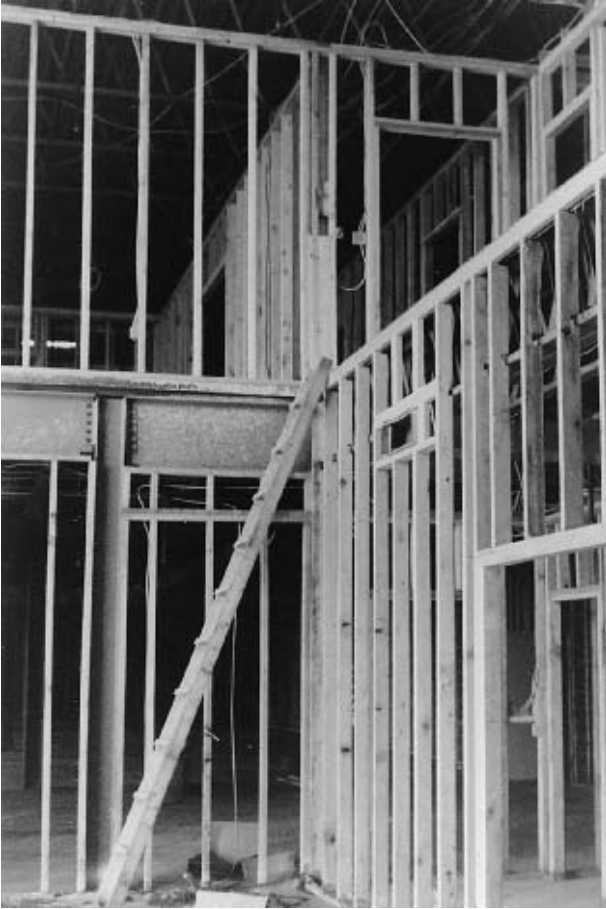
Fig. 12.1.11 A view of framing for the first- and second-story offices of a plant, with a roof beam and the steelwork supporting the second floor visible. (Source: VMA, Inc.)
