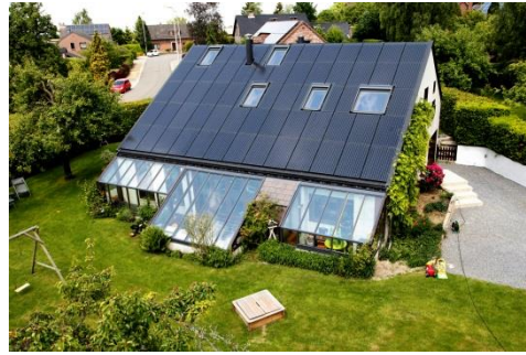
Tailor-made BIPV modules, ISSOL, Belgium
