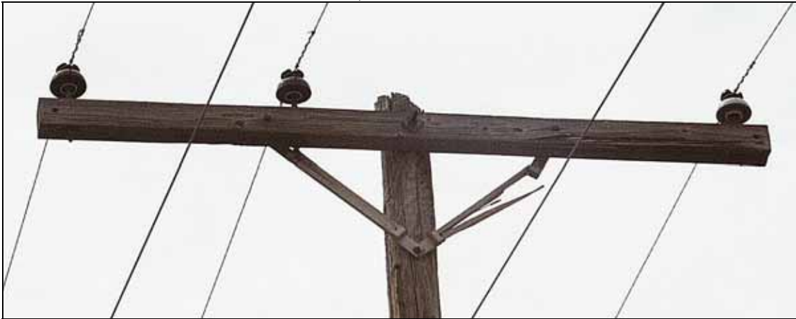
Figure 11 (Photo 05D6) Split wood brace (lightning damage), Circuit X96543, south of Lawrenceville
