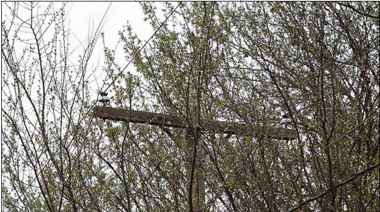
Figure 15 (Photo 05D15) Trees growing into primary, Circuit X96543, 9 th St. north of Harold St., St. Francisville
