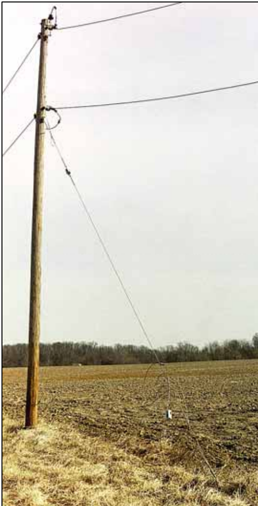
Figures 7 & 8 (Photos 05B19 & 05B18) Broken primary downguy (broken guy grip--possible lightning damage), Circuit V79594, northwest of Barrow
