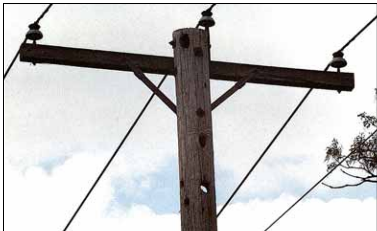
Figure 19 (Photo 05I16) Woodpecker hole through pole & other holes in pole, Circuit V23530, east of Detroit
