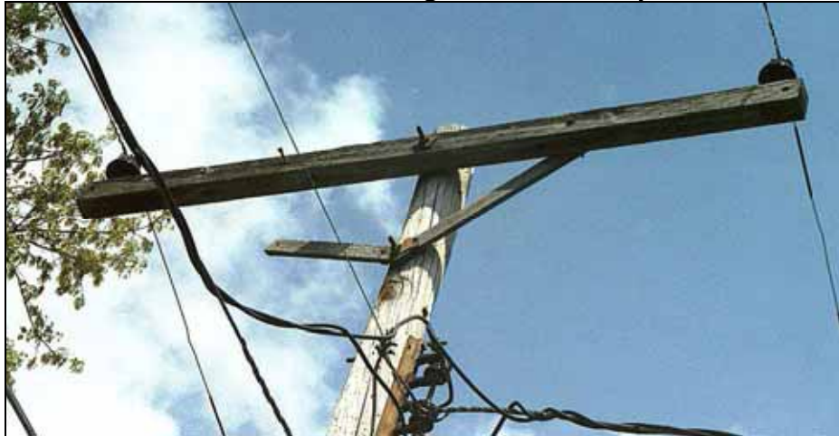
Figure 18 (Photo 05F14) Wood brace disconnected from crossarm, Circuit S47576, Orange St., Freeman Spur
