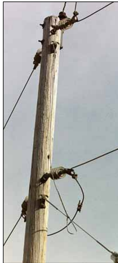
Figures 7 & 8 (Photos 05B19 & 05B18) Broken primary downguy (broken guy grip--possible lightning damage), Circuit V79594, northwest of Barrow
