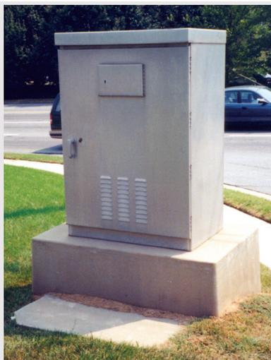
Many Departments of Transportation choose Hubbell traffic signal cabinet bases when they have projects requiring new and retrofit installations of traffic control cabinets. Hubbell traffic signal cabinet bases are less expensive than concrete to install, can be quickly installed by employees, can be relocated and can reduce potential injury and/or liability if struck by a vehicle.
