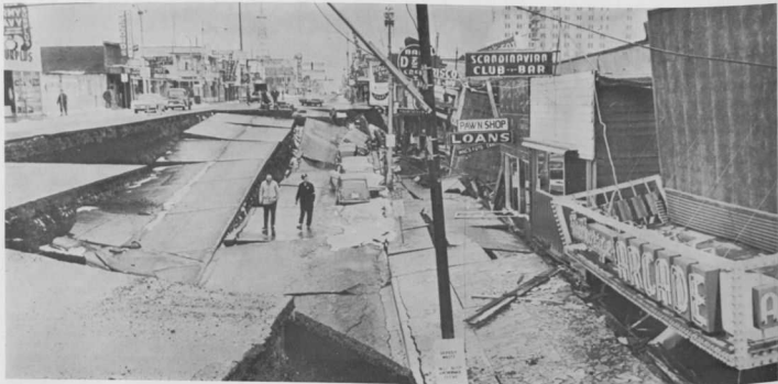
Wide World Photo These buildings, situated precisely over the fault which became the epicenter of the Good Friday earthquake in Alaska were among the most severely damaged in Anchorage. They are on Fourth Avenue and all were listed as total losses. This section fell some 10 feet below the other side of the fault.
