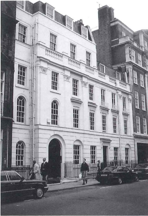
4. Nos.11 & 12 North Audley Street, built by Edward Sheperd c.1730, with later additions to No.12, on the left. Lord Ligonier's London home, and the 'War Office' during the Seven Years War. On the corner to the right, adjoining Grosvenor Square, is the house used by General Eisenhower as his 'War Office' during the Second World War. (Photograph by R.A. Buchanan)
