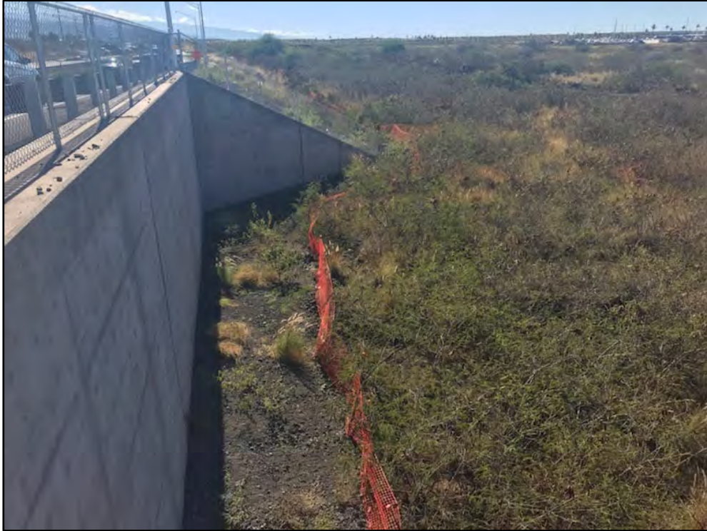
Figure 42. Photo showing southern portion of Retaining Wall A-1; view to southwest
