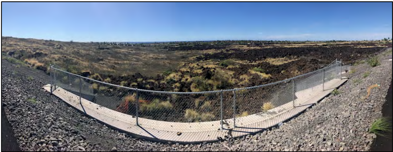
Figure 45. Panoramic photo of Retaining Wall E; view to west
