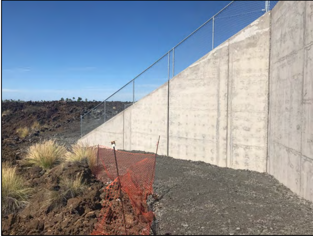
Figure 44. Photo showing northern portion of Retaining Wall E; view to northwest
