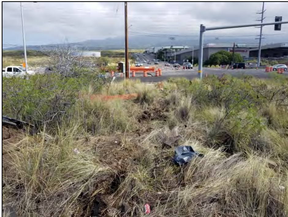
Figure 68. Photo depicting the extent of damage caused by the vehicle accident at the Hinalani intersection; view to east
