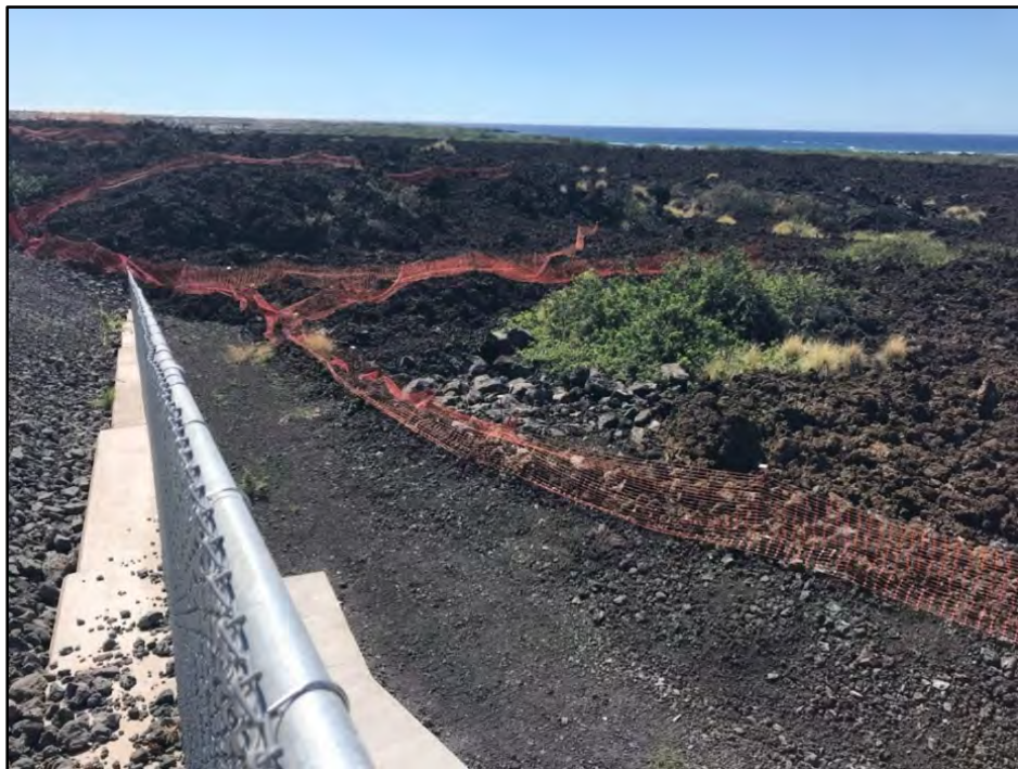
Figure 41. Photo of southern portion of Retaining Wall A with SIHP # -28783 visible in background; view to southwest
