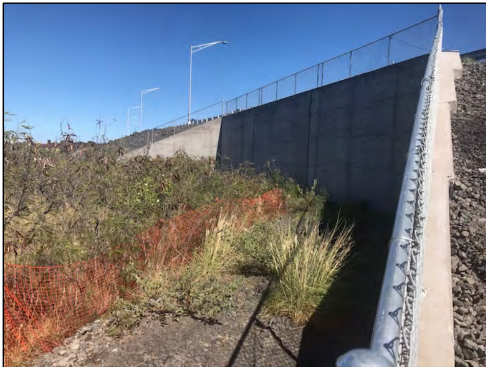
Figure 43. Photo of Retaining Wall A-1; view to northeast
