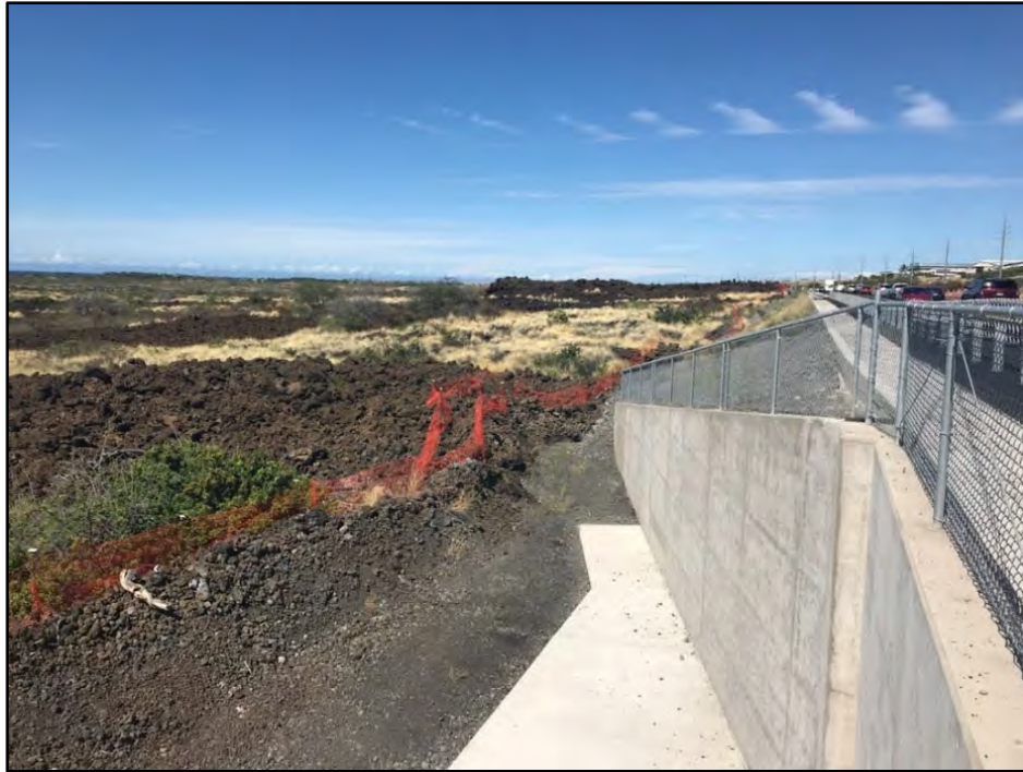
Figure 40. Photo showing northern portion of Retaining Wall A; view to northwest
