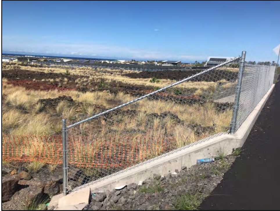
Figure 46. Photo of southern portion of Retaining Wall F; view to northwest
