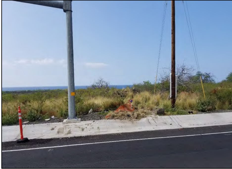
Figure 67. Photo showing the location of the vehicle accident on the makai side of the Hina Lani Street and Queen Ka'ahumanu Highway intersection; note the breached interim construction fencing; view to west
