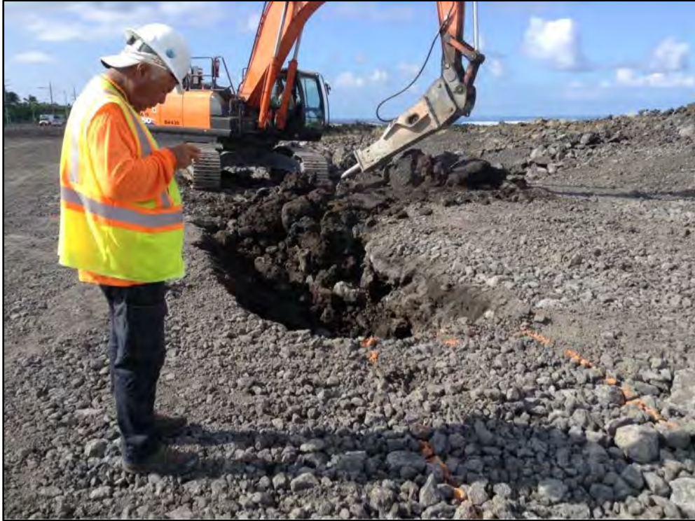
Figure 56. Photo showing the location of Lava Tube Breach #1; view to southwest
