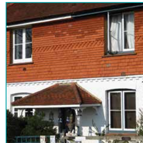
Barnside Cottages, Ripley Lane
