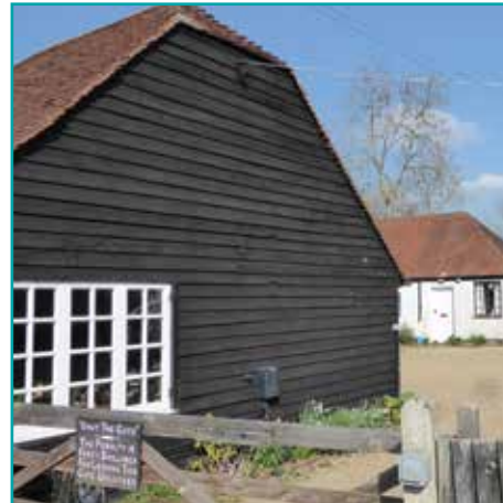
Outbuilding within the curtilage of Barcombe Farm
