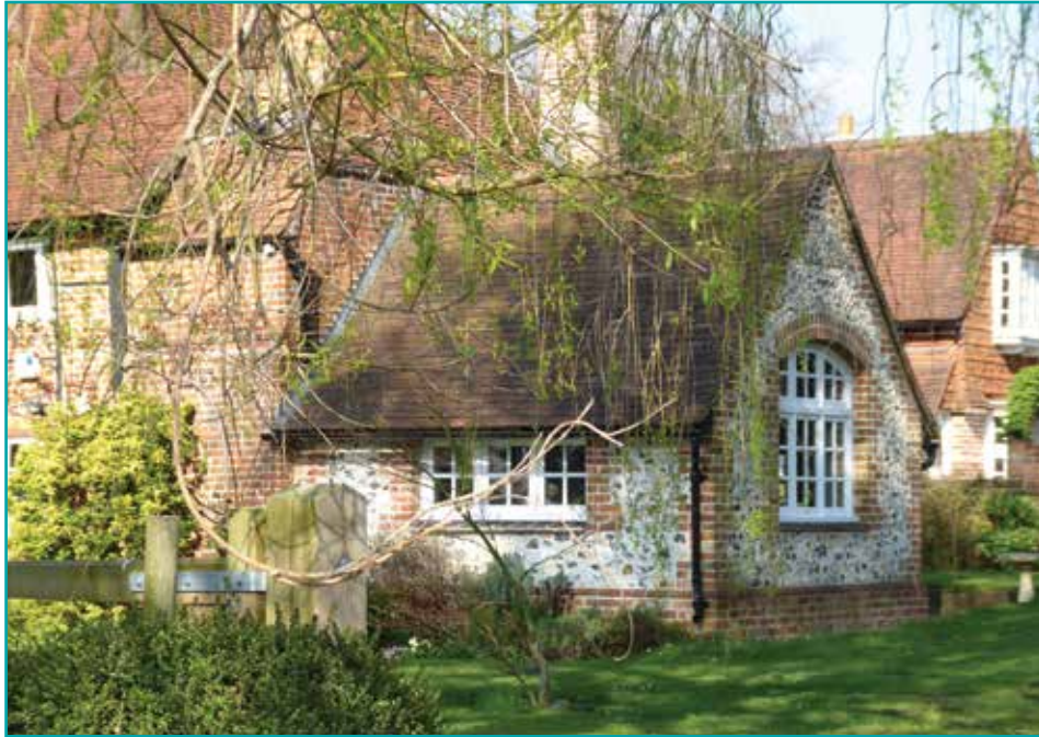
Single storey extension of flint construction seen at Pincott Farm House, Pincott Lane
