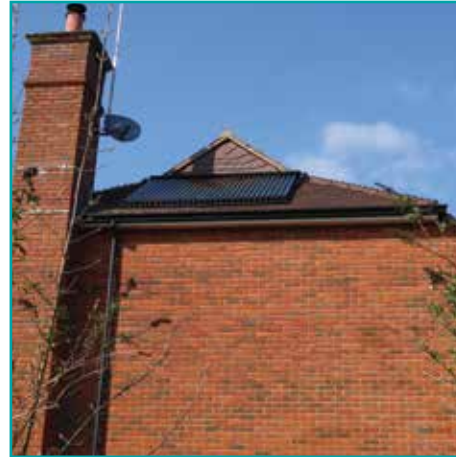
Modern brick development
