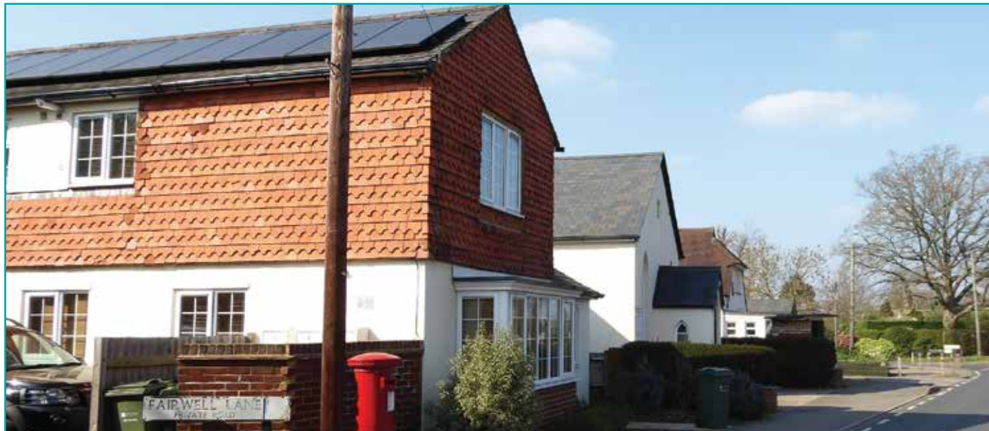
No 95, The Street exhibiting a patterned hanging tile detail to its upper storey
