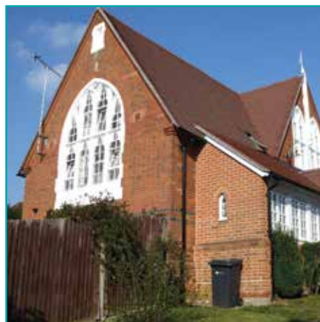
Former St Mary's School
