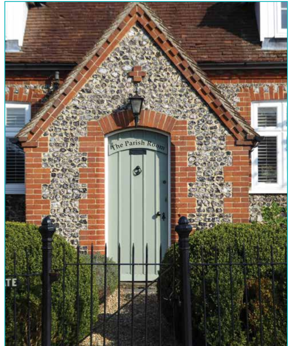
Enclosed porch, The Parish Room, The Street
