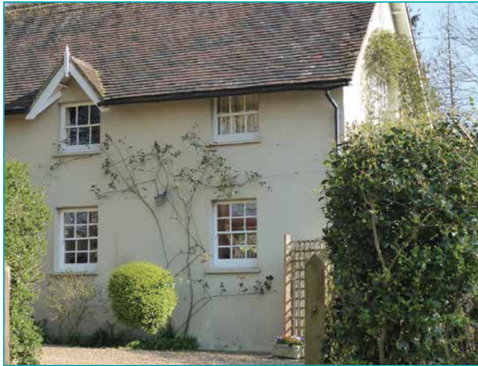
Sliding sash windows of timber construction at Brinkwells, Pincott Lane
