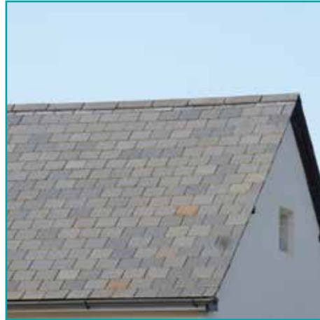
Machine formed 'slate' roof covering the Methodist Chapel
