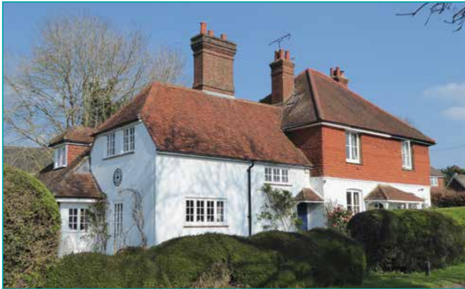
Barnside Cottages, Ripley Lane
