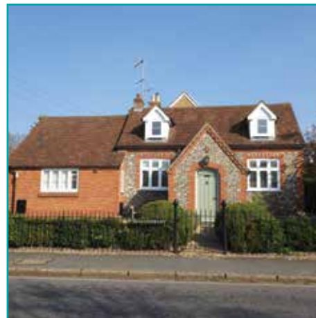
The Parish Rooms
