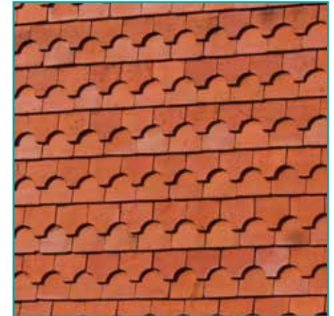
Alternating layers of fishtail and plain tiles provides additional visual interest
