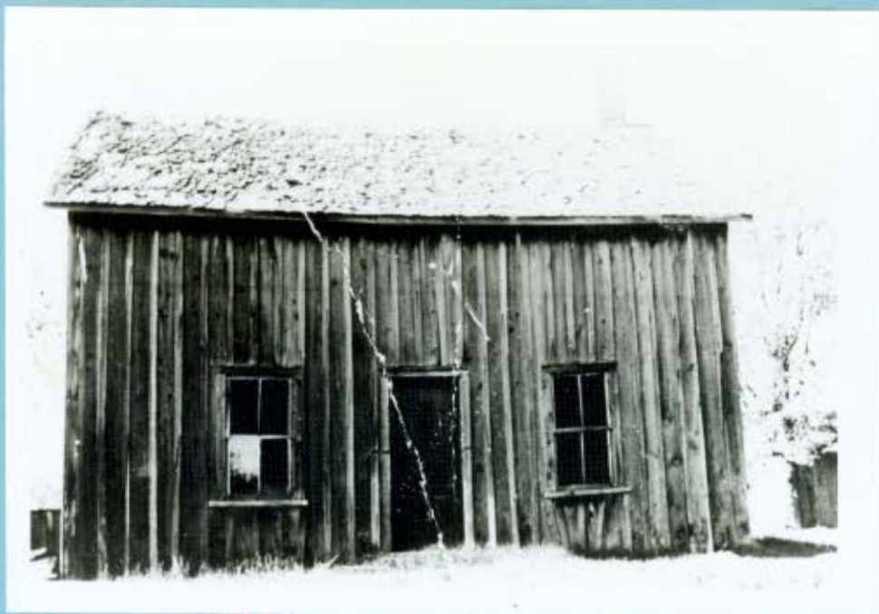
Old house on lot 42 con. 3 before it was remodeled.
