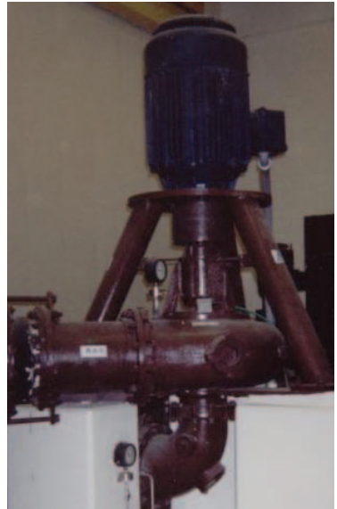
Model NSWV with Tri-base on RAS service.
