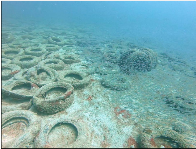
Photo C-25. Large concentration of loose tires near Site D2, north of Osborne Tire Reef northern boundary.
